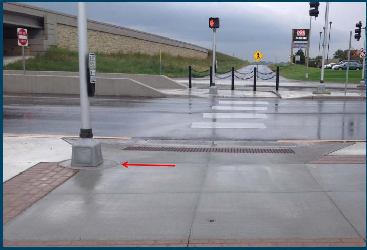
New Pedestal Foundations shall be constructed flush to within 1/4" of Landing.
