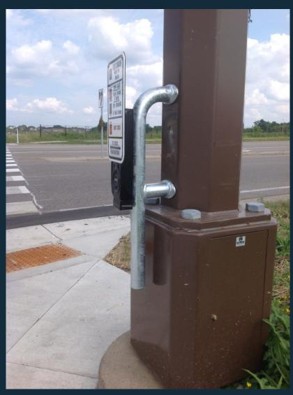
Signal pole Foundations: The APS push button shall meet the vertical horizontal and crosswalk skew requirements.
