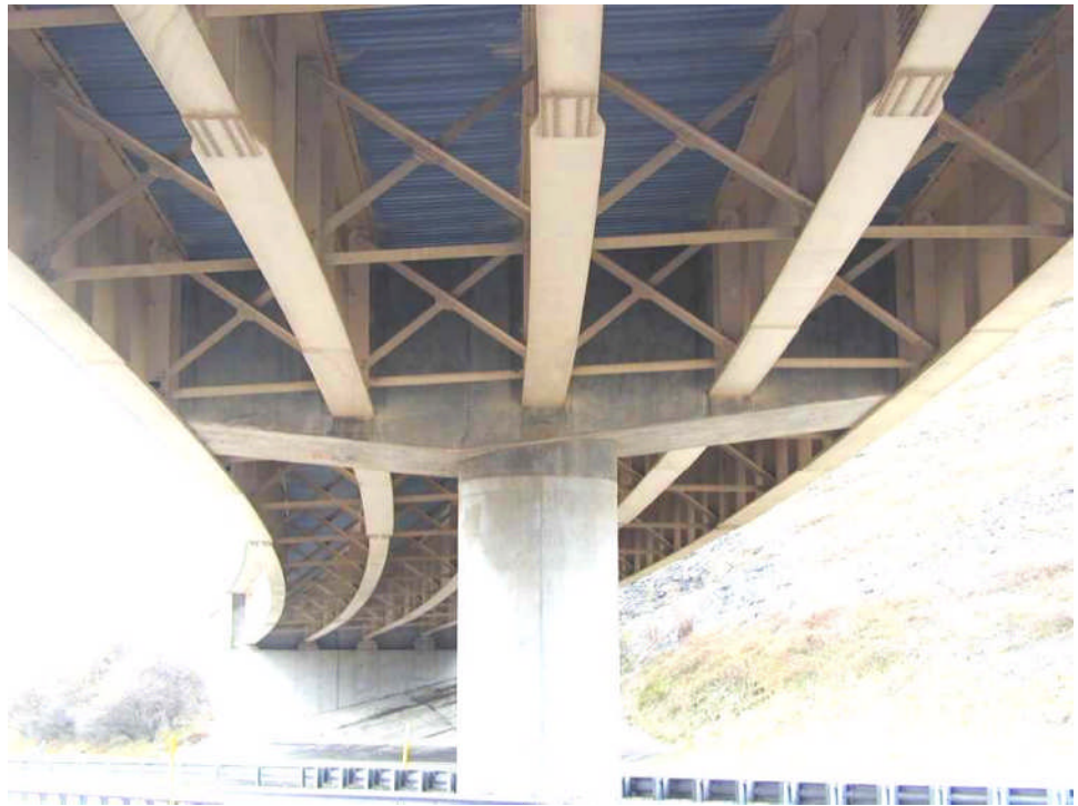
Figure 12.2.12 Integral Concrete Pier and Pier Cap
