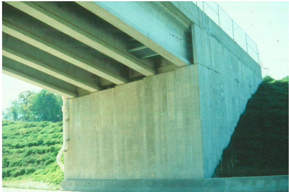
Figure 12.1.4 Full Height Abutment
