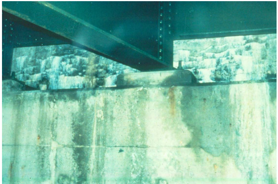
Figure 12.1.33 Cracking and Efflorescence in Abutment Backwall
