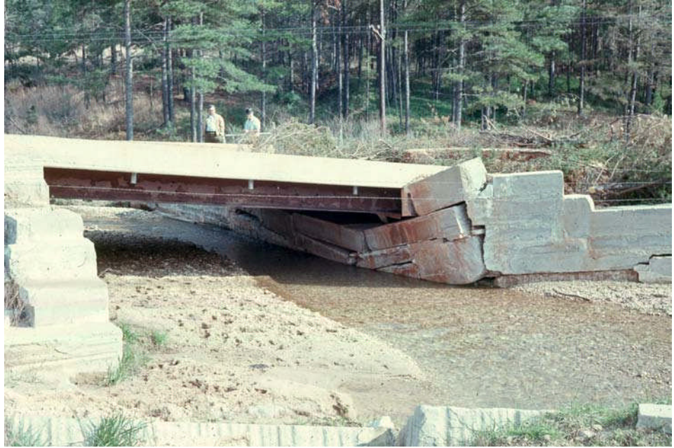
Figure 12.1.50 Abutment with Undermining due to Scour
