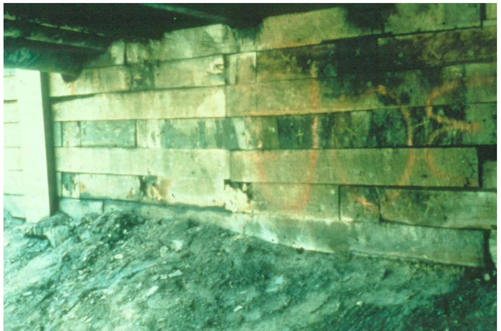
Figure 12.1.36 Decay caused by insects in Timber Abutment
