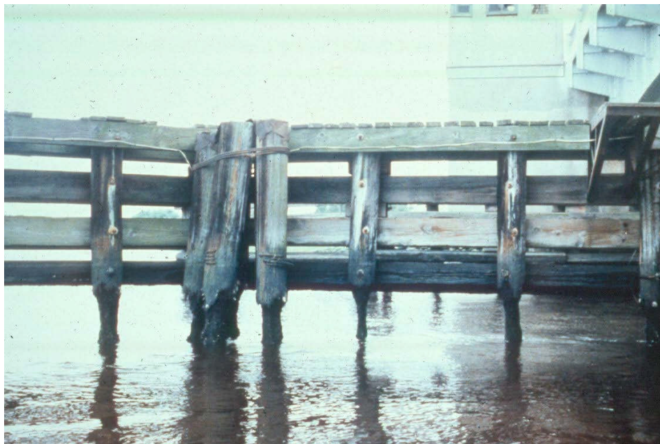
Figure 12.2.54 Timber Fender System with Deteriorated Piles
