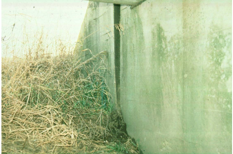
Figure 12.1.49 Rotational Movement at Concrete Wingwall
