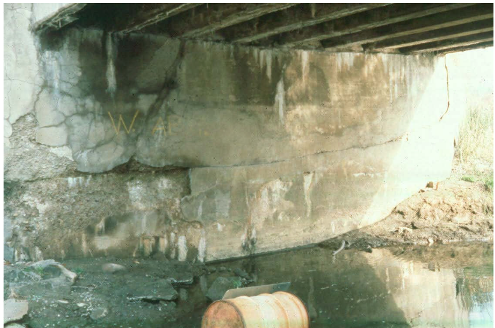
Figure 12.1.13 Plain Unreinforced Concrete Gravity Abutment
