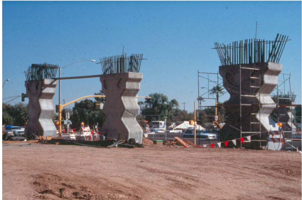
Figure 12.2.13 Reinforced Concrete Piers under Construction
