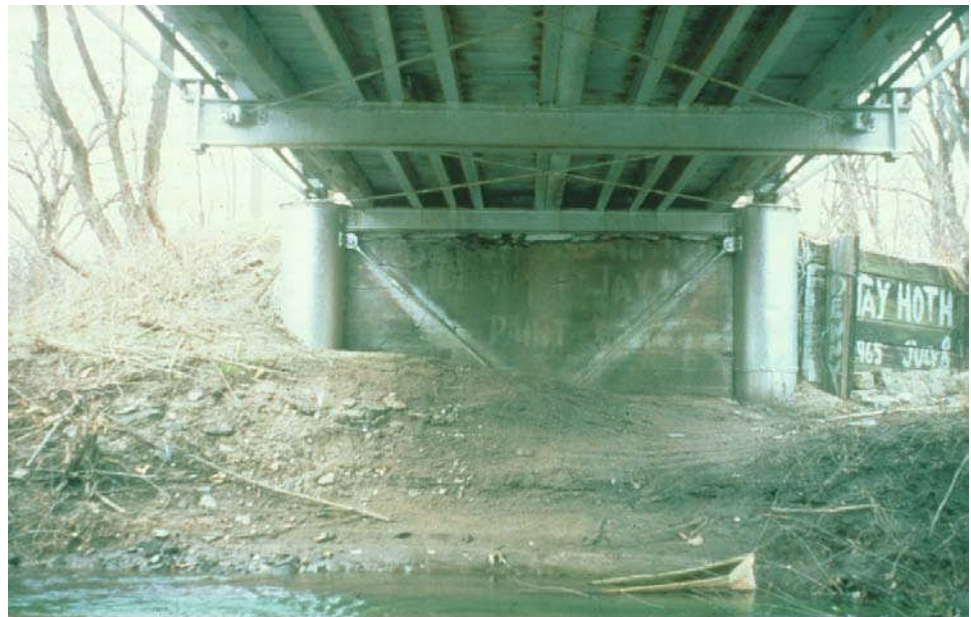
Figure 12.1.35 Steel Abutment
