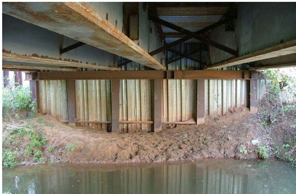
Figure 12.1.17 Steel Abutment
