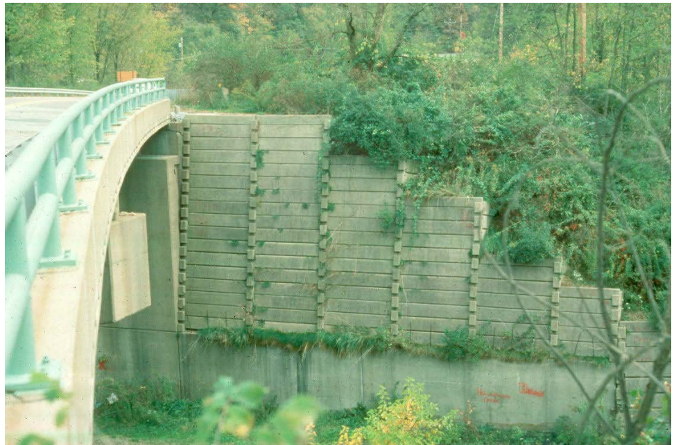
Figure 12.1.24 Straight Wingwall
