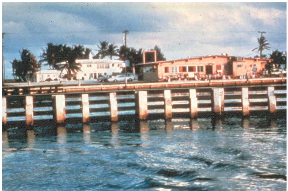
Figure 12.2.29 Fender System
