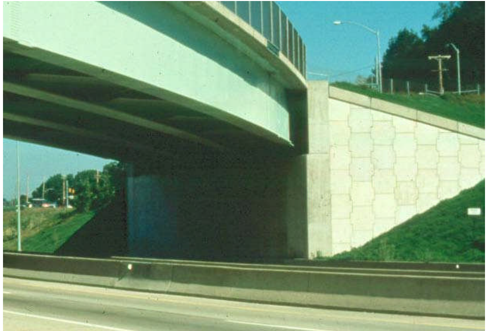
Figure 12.1.28 Independent MSE Wingwall
