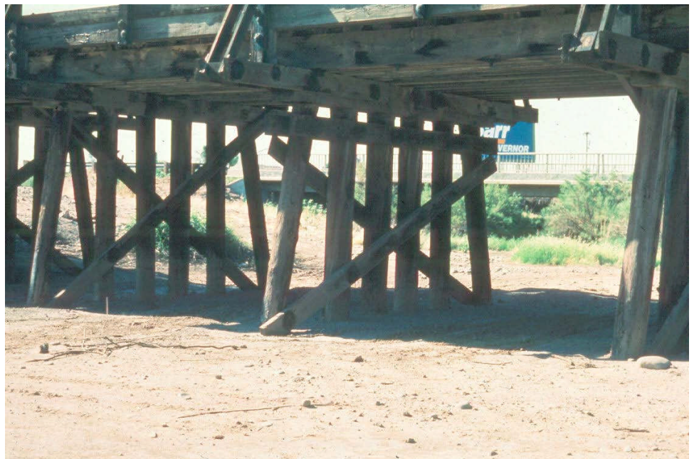
Figure 12.2.16 Timber Pile Bent
