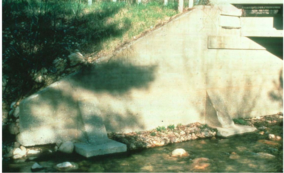
Figure 12.1.52 Scour and Possible Undermining of Concrete Wingwall
