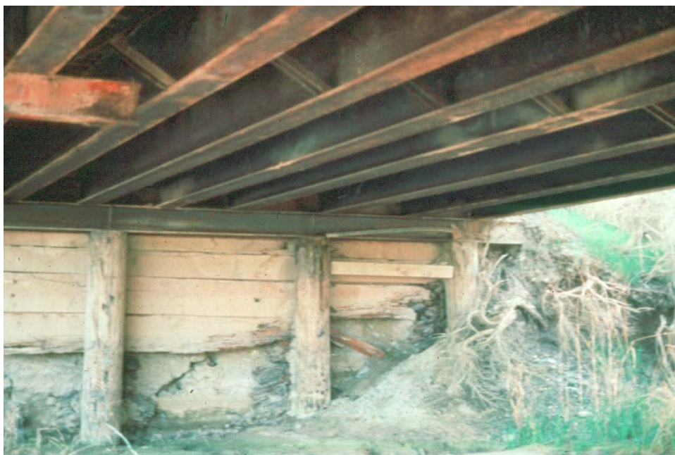
Figure 12.1.38 Decayed Lagging and Abrasion Caused by Scour at a Timber Pile Bent Abutment
