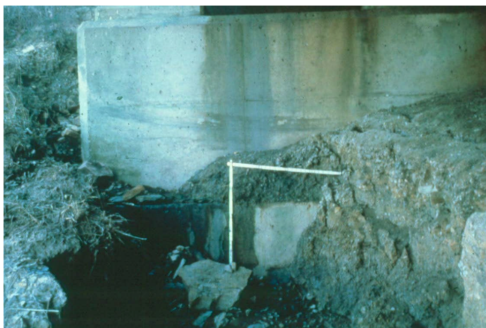
Figure 12.1.45 Erosion at Abutment Exposing Footing
