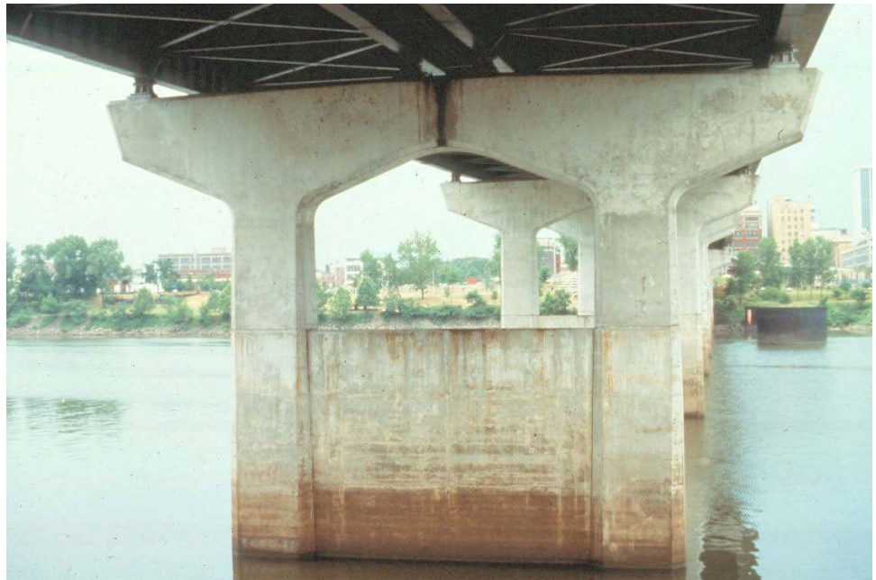
Figure 12.2.22 Cantilevered Piers Joined by a Web Wall
