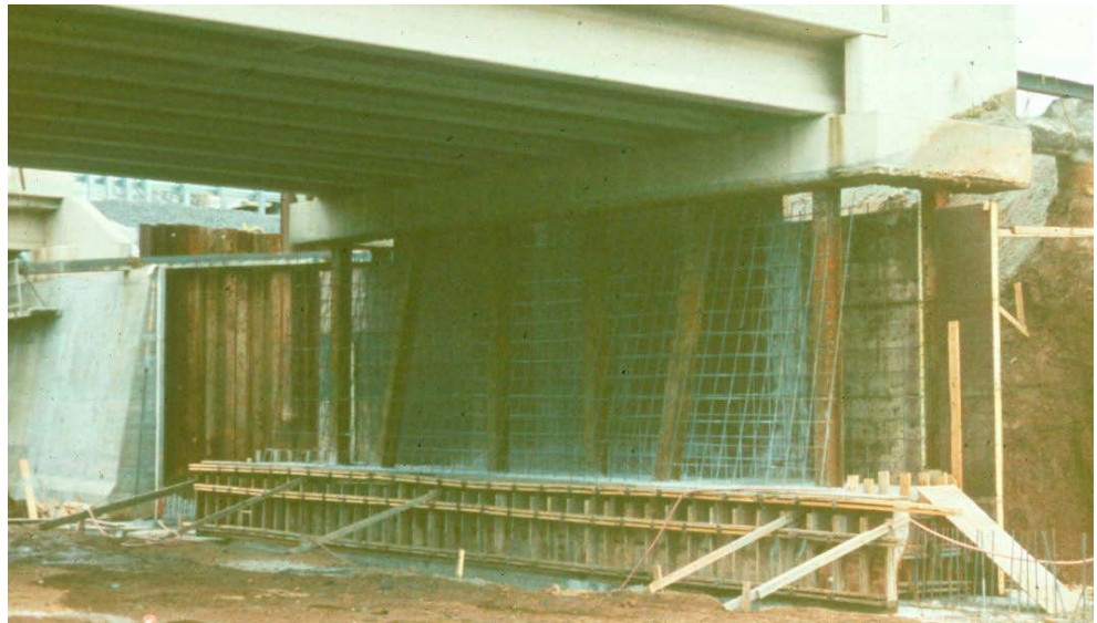
Figure 12.1.22 Stub Abutment on Piles with Piles Exposed
