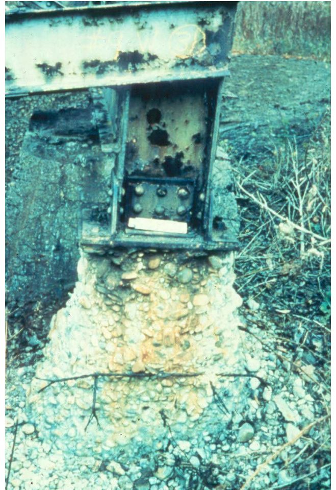
Figure 12.2.35 Deterioration of Steel Bent Leg
