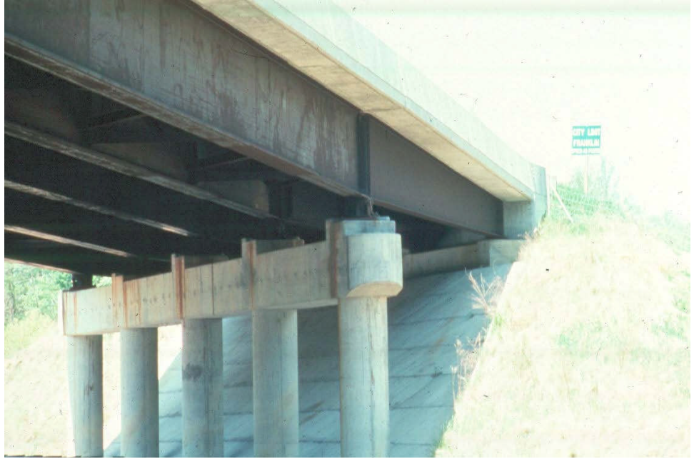
Figure 12.2.8 Column Bent or Open Bent
