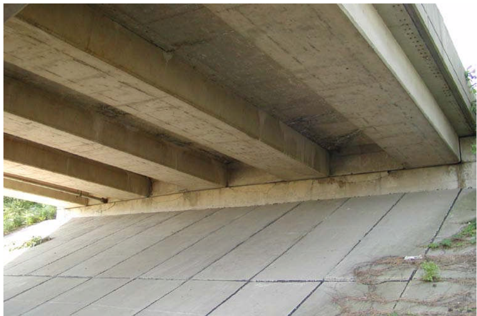
Figure 12.1.5 Stub Abutment
