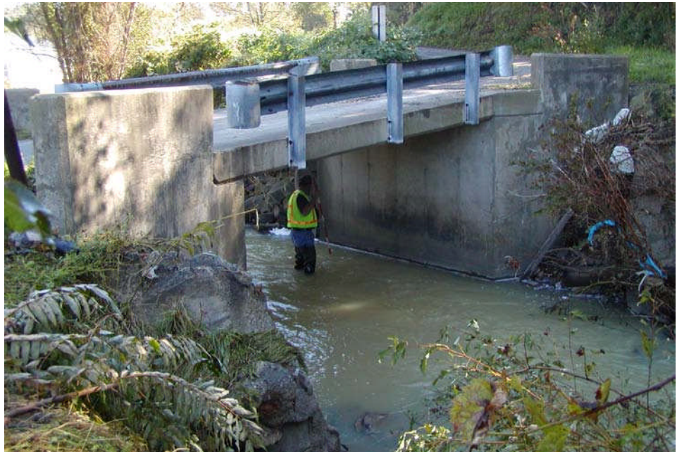
Figure 12.1.51 Inspector Checking for Scour
