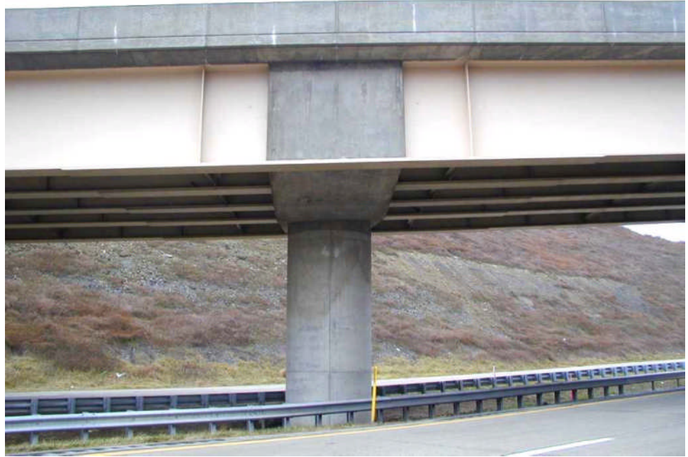
Figure 12.2.11 Integral Concrete Pier and Pier Cap
