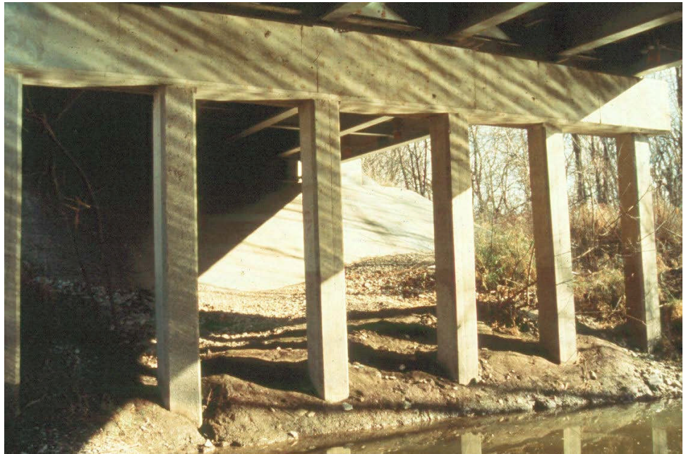
Figure 12.2.9 Concrete Pile Bent
