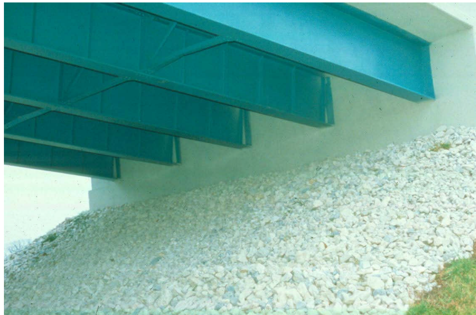
Figure 12.1.8 Integral Abutment
