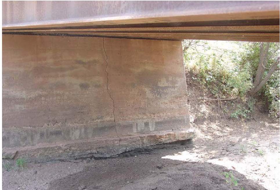
Figure 12.1.41 Crack in Abutment due to Settlement
