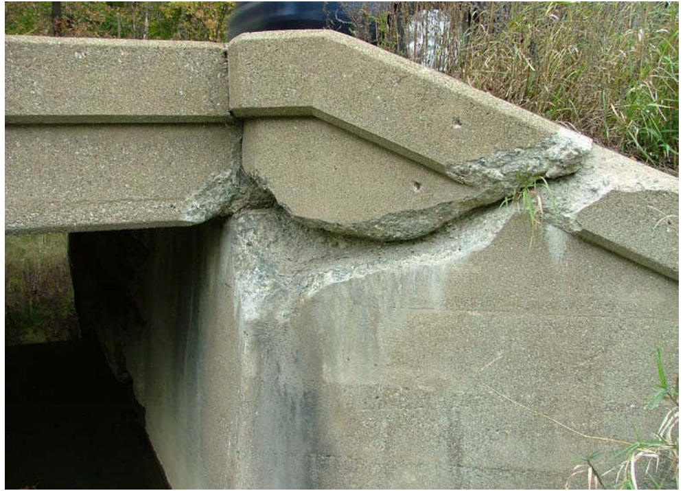
Figure 12.1.32 Spalled Concrete Wingwall
