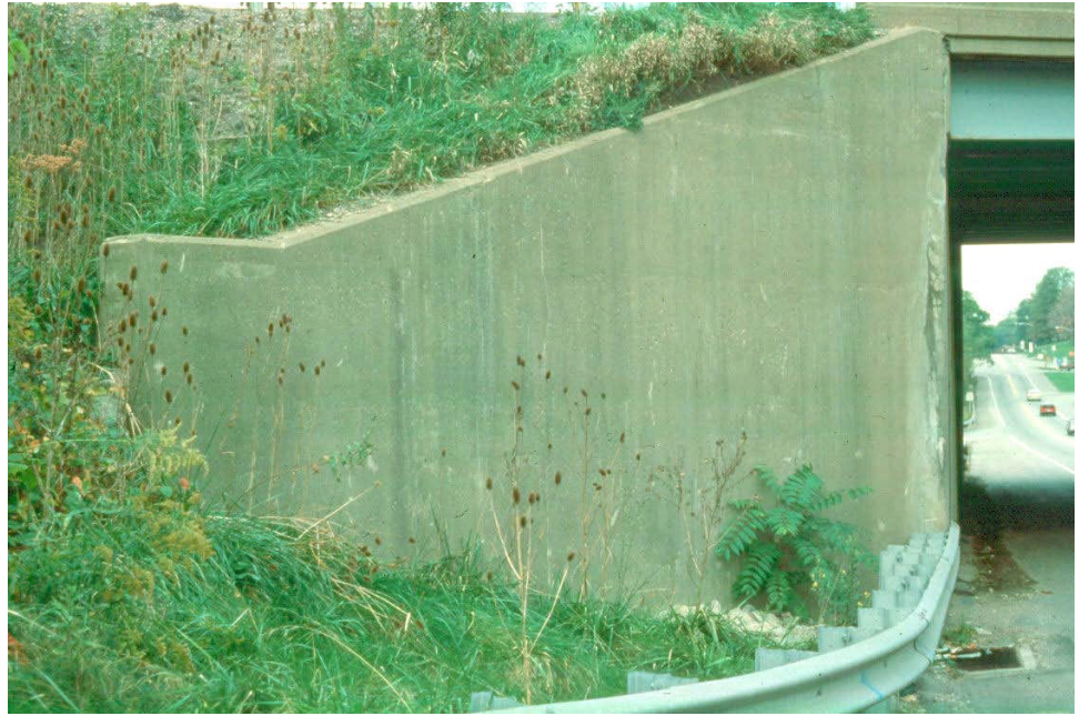
Figure 12.1.23 Typical Wingwall
