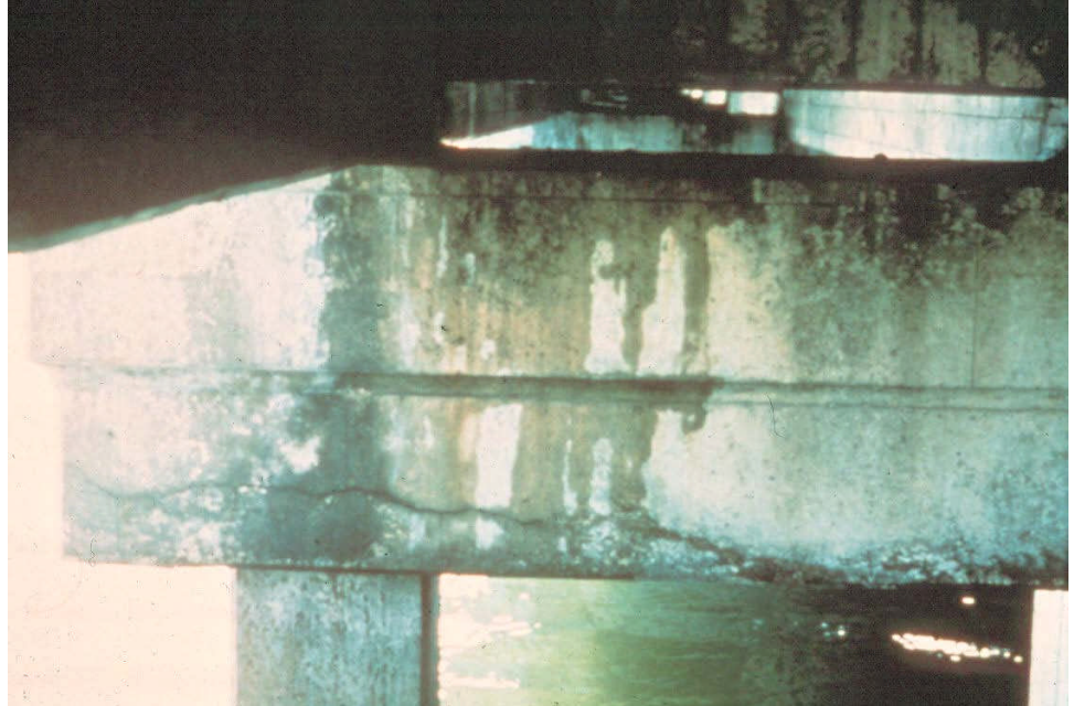
Figure 12.2.31 Crack in Concrete Bent Cap
