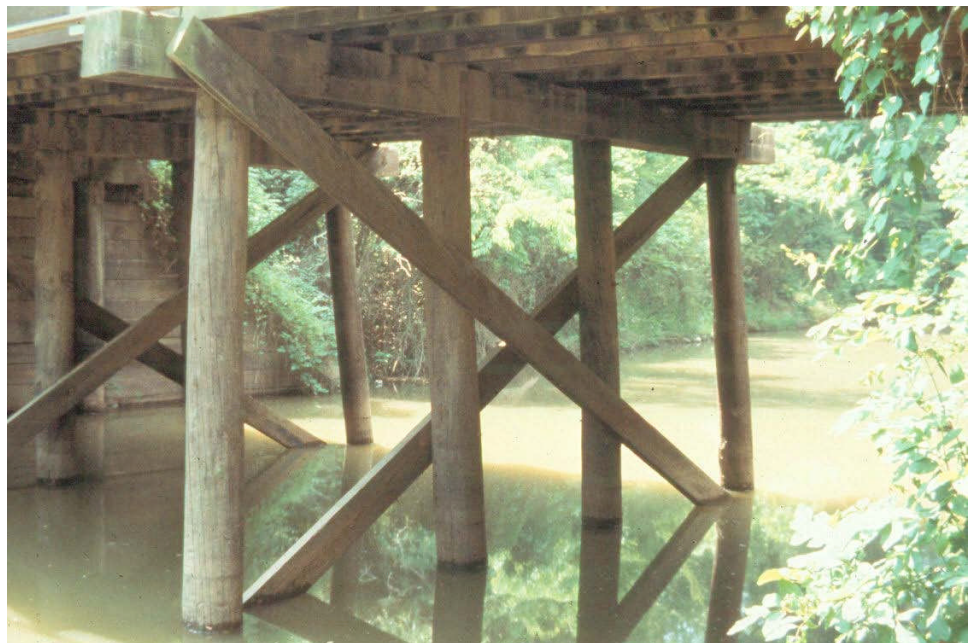
Figure 12.2.39 Timber Bent Columns in Water
