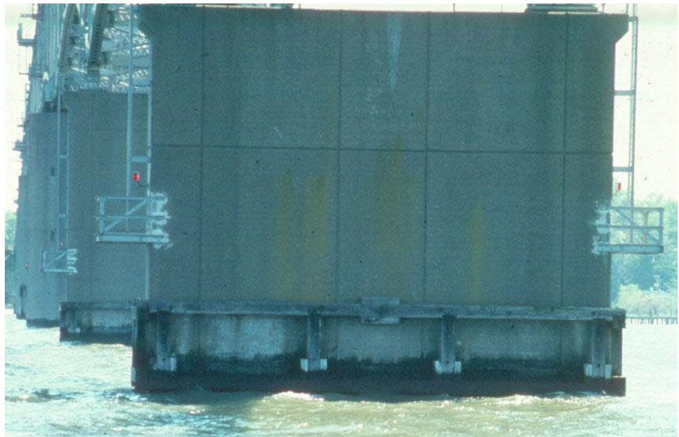
Figure 12.2.53 Steel Fender
