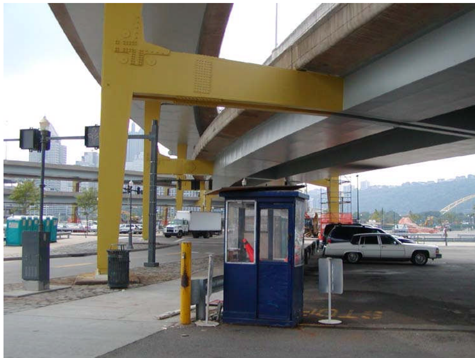
Figure 12.2.51 Fracture Critical Steel Bent
