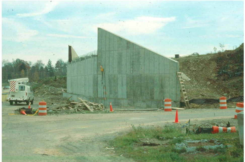
Figure 12.1.14 Reinforced Concrete Cantilever Abutment
