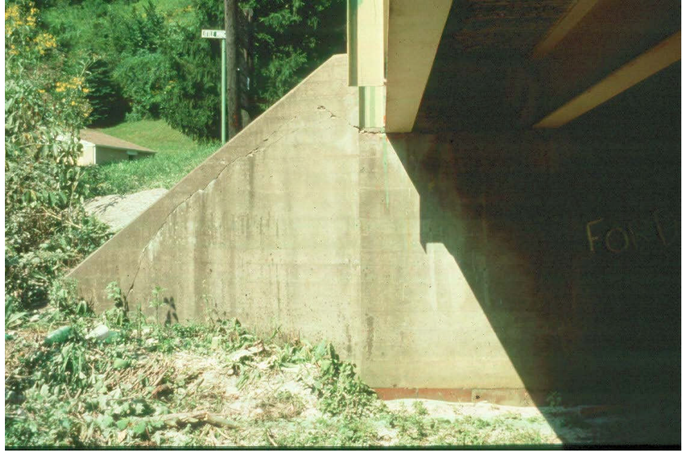
Figure 12.1.25 Flared Wingwall
