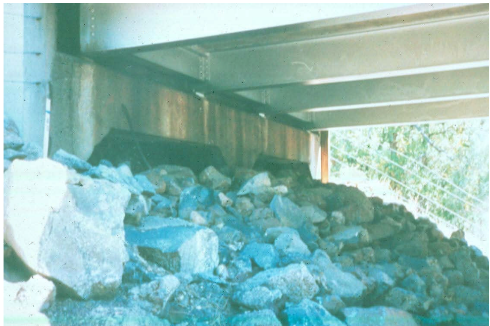
Figure 12.1.6 Open Abutment
