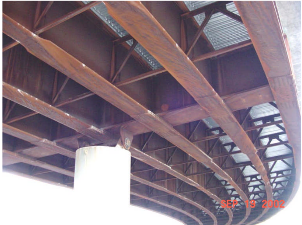
Figure 12.2.10 Concrete Pier with Integral Steel Pier Cap
