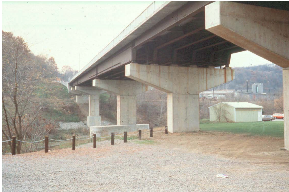
Figure 12.2.7 Cantilever Pier
