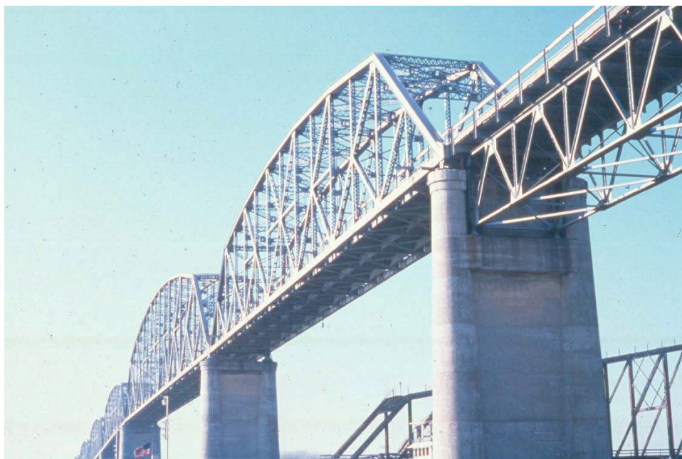
Figure 12.2.5 Column Pier with Web Wall
