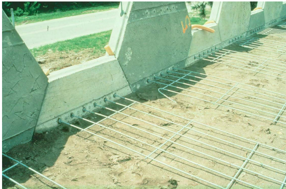
Figure 12.1.10 Mechanically Stabilized Earth Wall Under Construction
