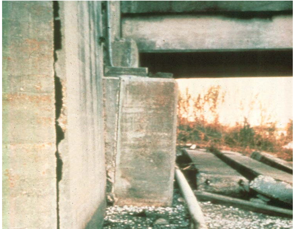
Figure 12.1.47 Rotational Movement at Abutment
