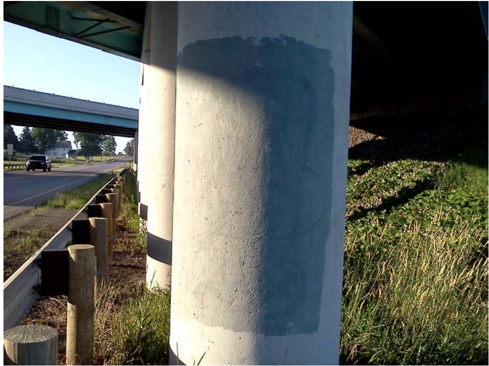
Figure 12.2.50 Repaired Concrete Column Bent
