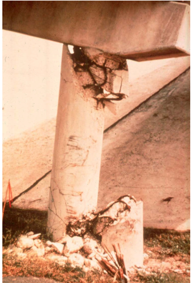
Figure 12.2.33 Collision Damage to Concrete Pier Column
