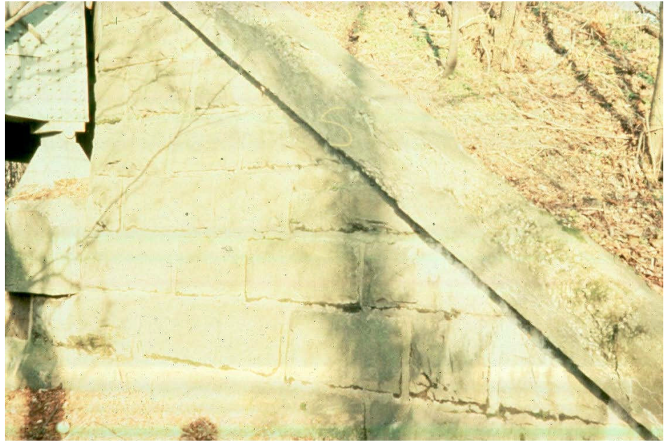
Figure 12.1.29 Masonry Wingwall
