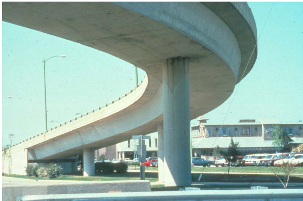
Figure 12.2.3 Column Pier
