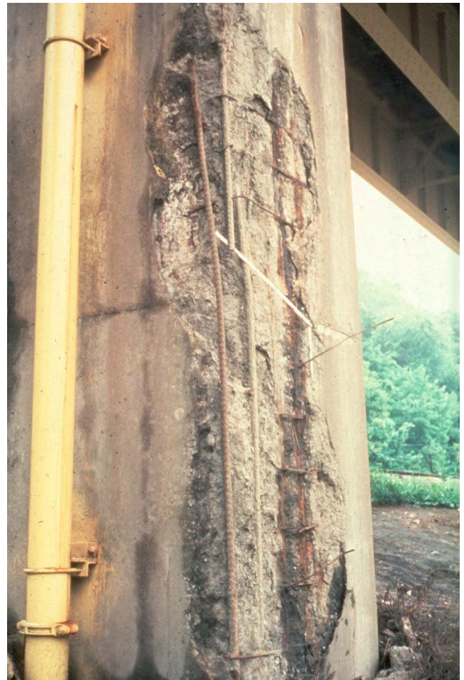
Figure 12.2.30 Concrete Spalling due to Contaminated Drainage
