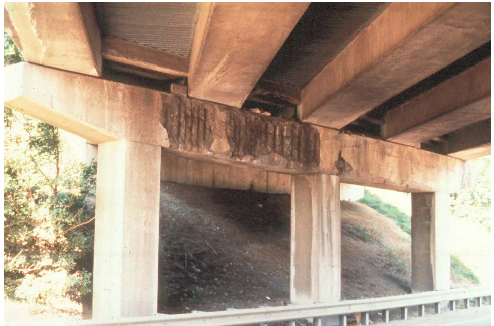
Figure 12.2.32 Concrete Spalling on Bent Cap
