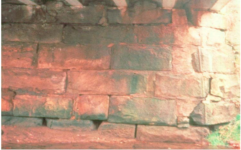
Figure 12.1.34 Stone Masonry Abutment with Deteriorated Joints
