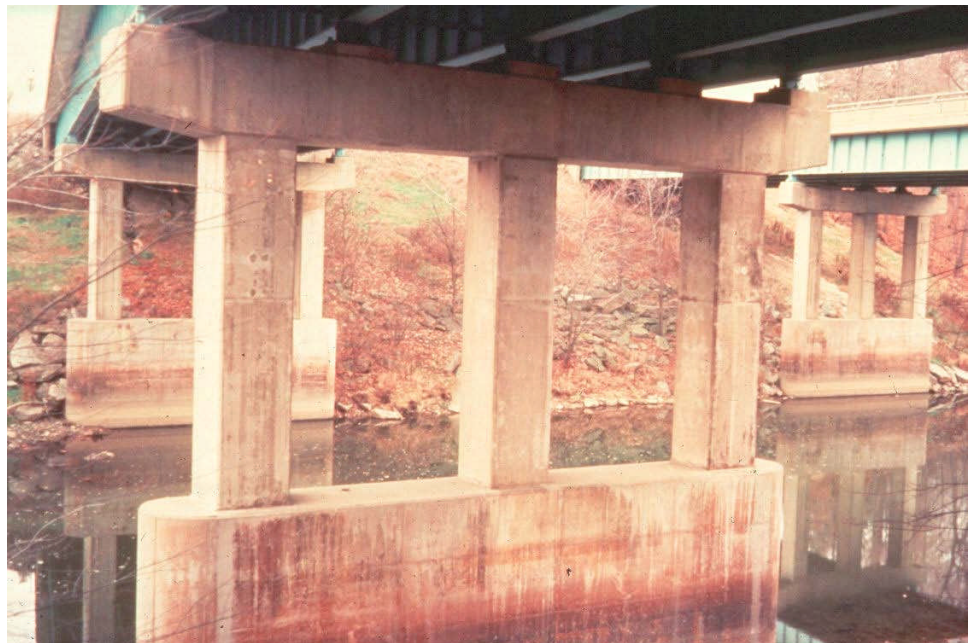
Figure 12.2.25 Collision Wall
