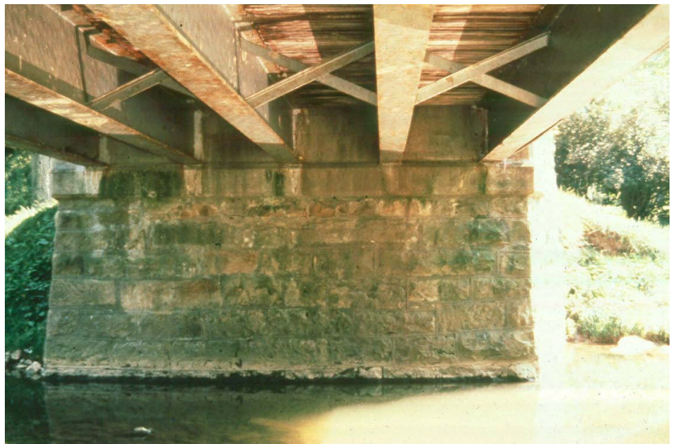
Figure 12.1.15 Stone Masonry Gravity Abutment
