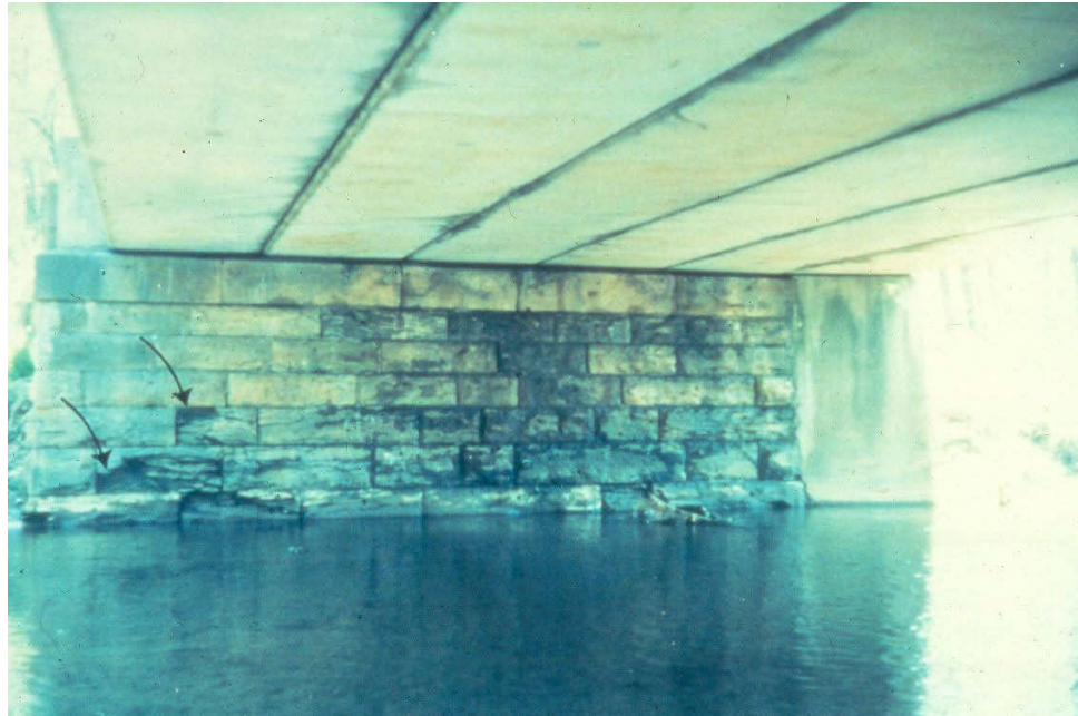
Figure 12.2.34 Deteriorated and Missing Stone at Masonry Pier
