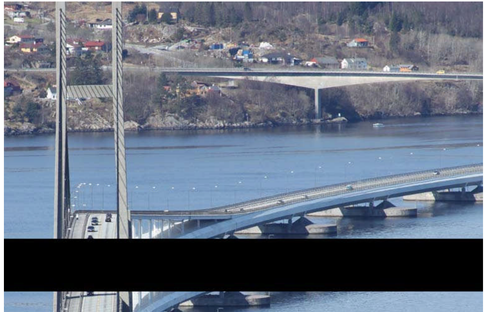
Figure 16.3.9 Bridge Constructed with Separate Pontoons
