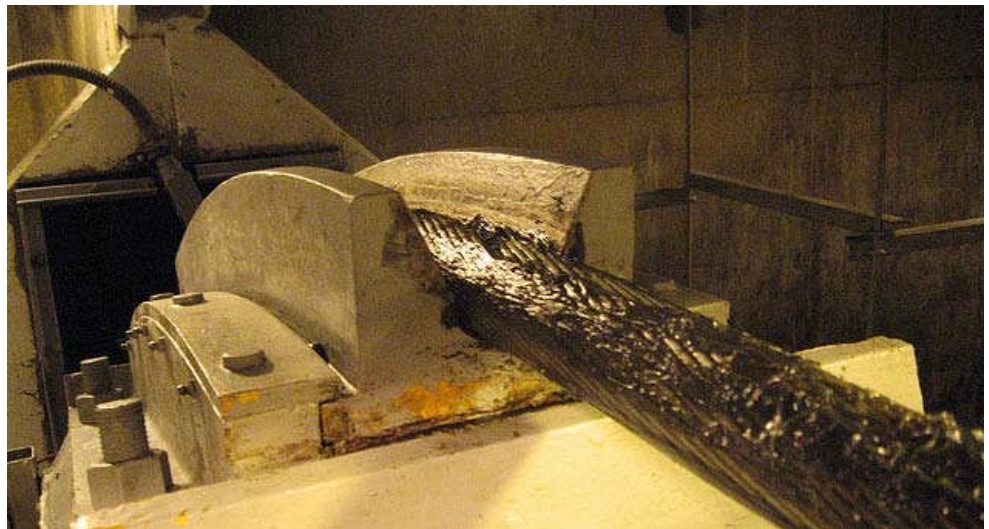
Figure 16.3.11 Anchor Cable Saddle
