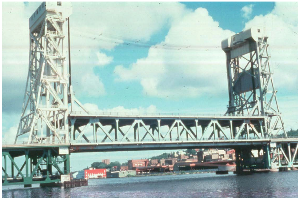
Figure 16.2.33 Concrete Counterweight on a Vertical Lift Bridge
