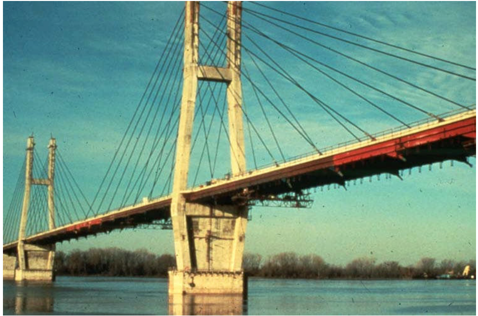
Figure 16.1.30 Double Vertical Plane Cable System
