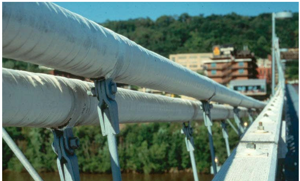
Figure 16.1.12 Cable Wrapping on the Wheeling Suspension Bridge
