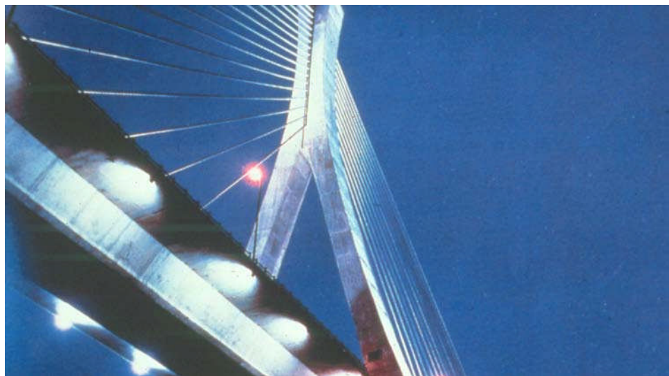
Figure 16.1.29 Single Vertical Plane Cable System
