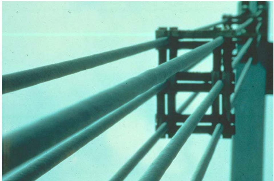
Figure 16.1.24 Cable Tie Damper System
