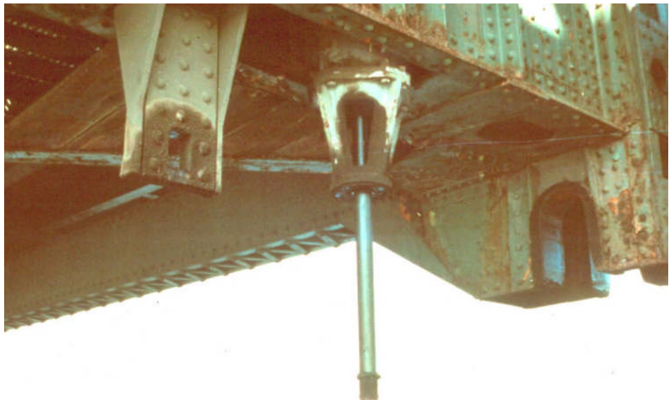
Figure 16.2.27 Air Buffer
