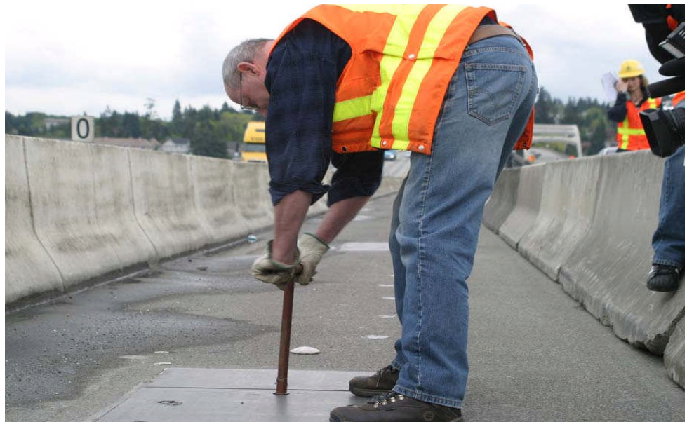
Figure 16.3.16 Inspector Opening Pontoon Access Hatch
