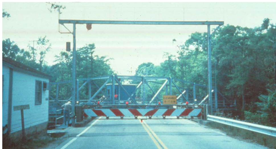
Figure 16.2.35 Traffic Barrier
