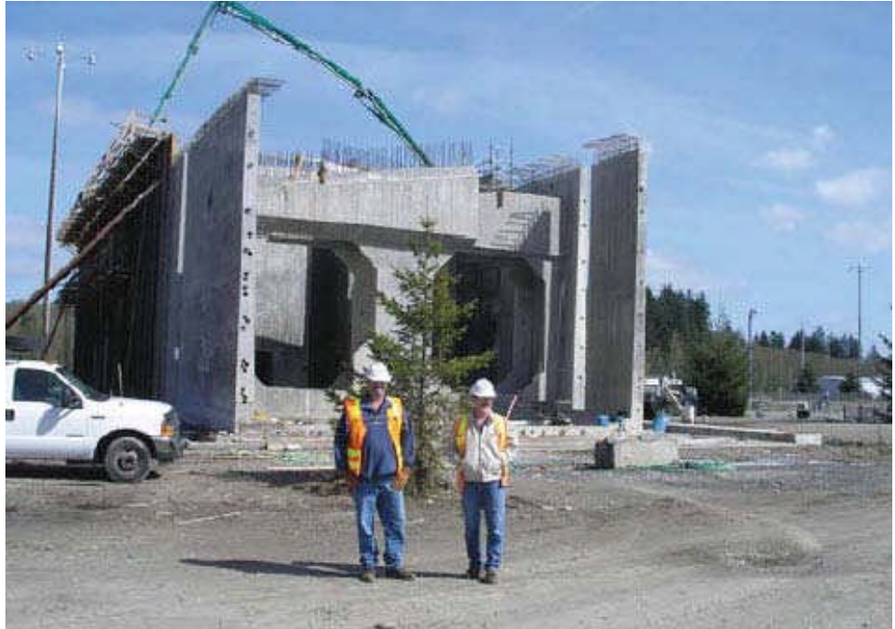
Figure 16.3.5 Concrete Pontoons Under Construction
