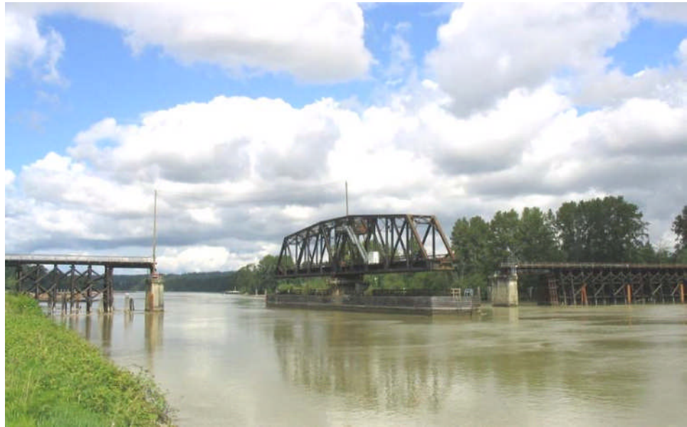
Figure 16.2.4 Center-Bearing Swing Bridge
