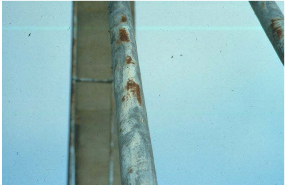
Figure 16.1.44 Corrosion of Steel Sheathing
