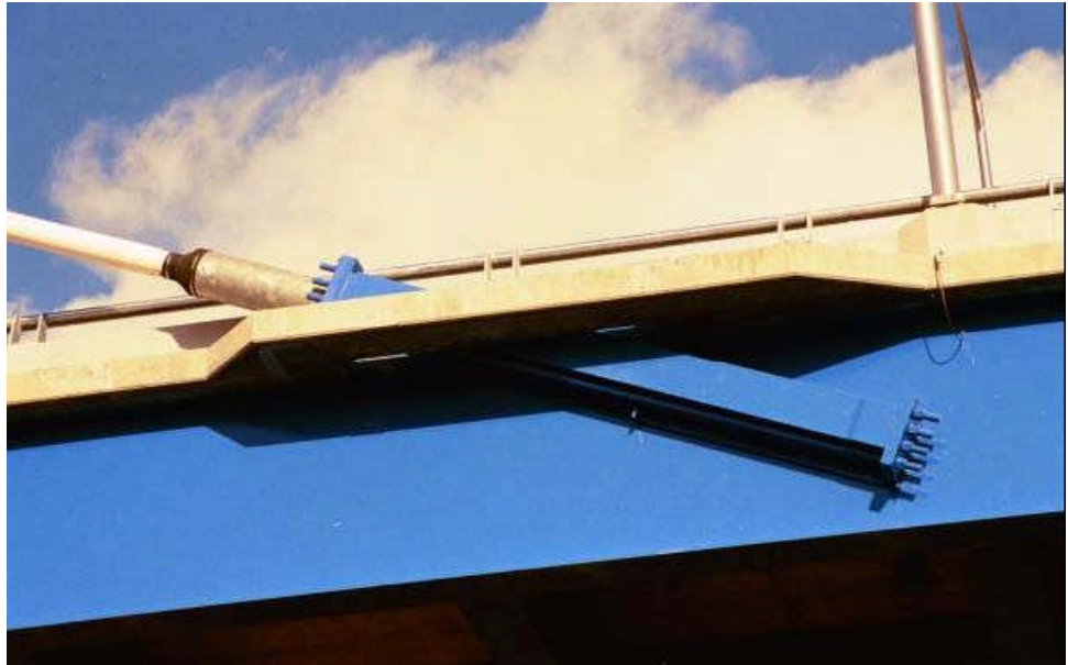
Figure 16.1.33 Cable Deck Anchorage
