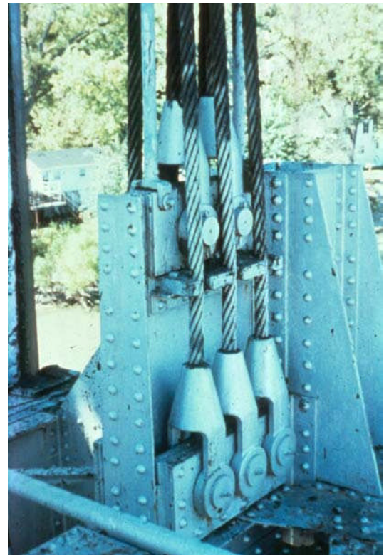
Figure 16.2.51 Wire Rope Sockets and Fittings
