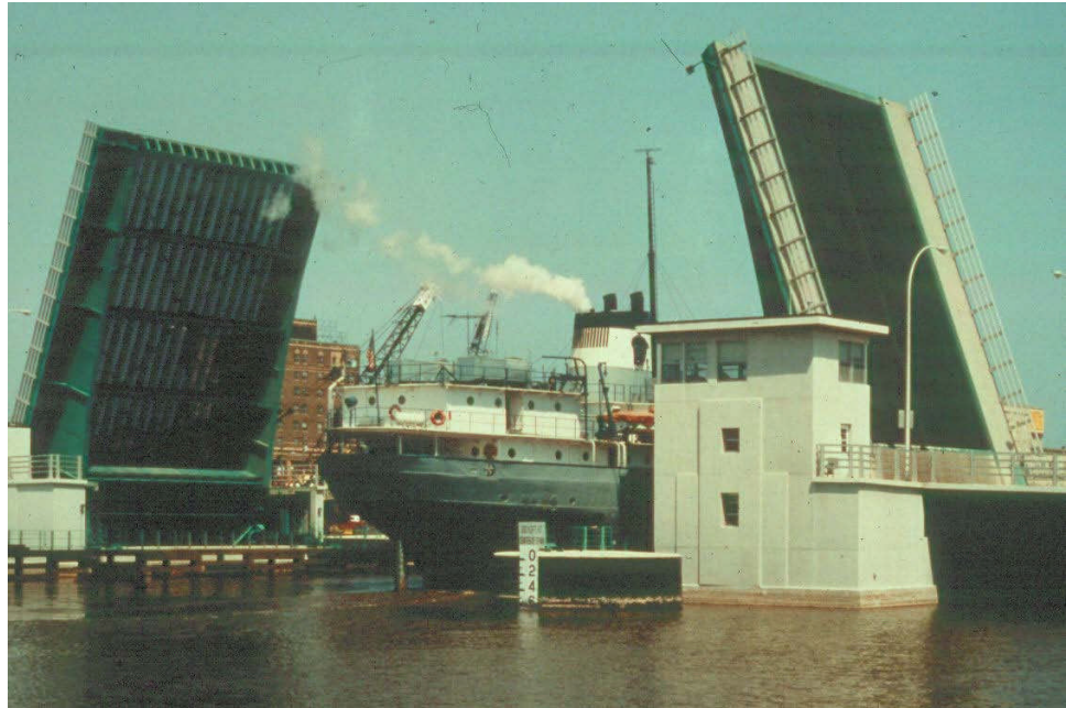
Figure 16.2.9 Double-Leaf Rolling Lift Bascule
