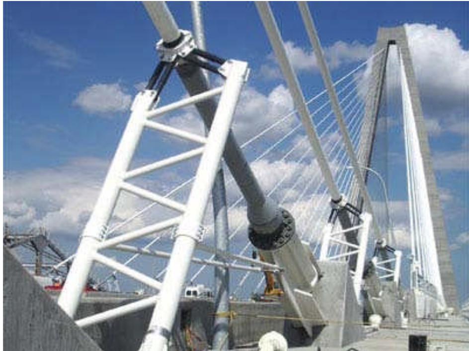
Figure 16.1.48 Shock Absorber Damper System
