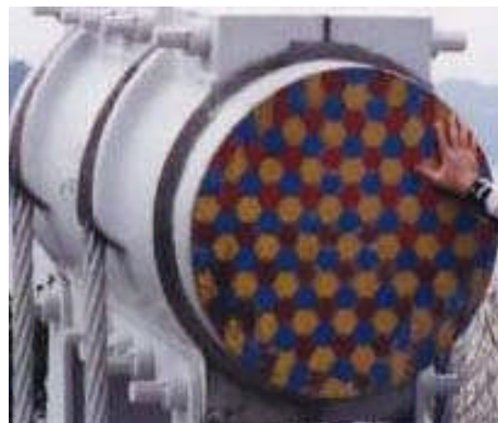
Figure 16.1.8 Parallel Strand Cable
