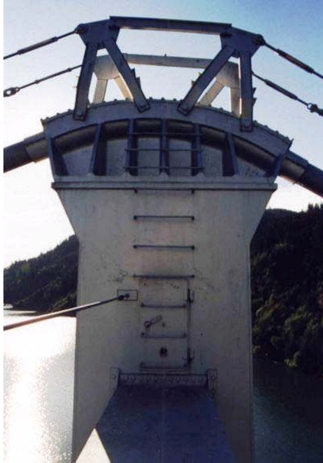
Figure 16.1.32 Cable Saddle
