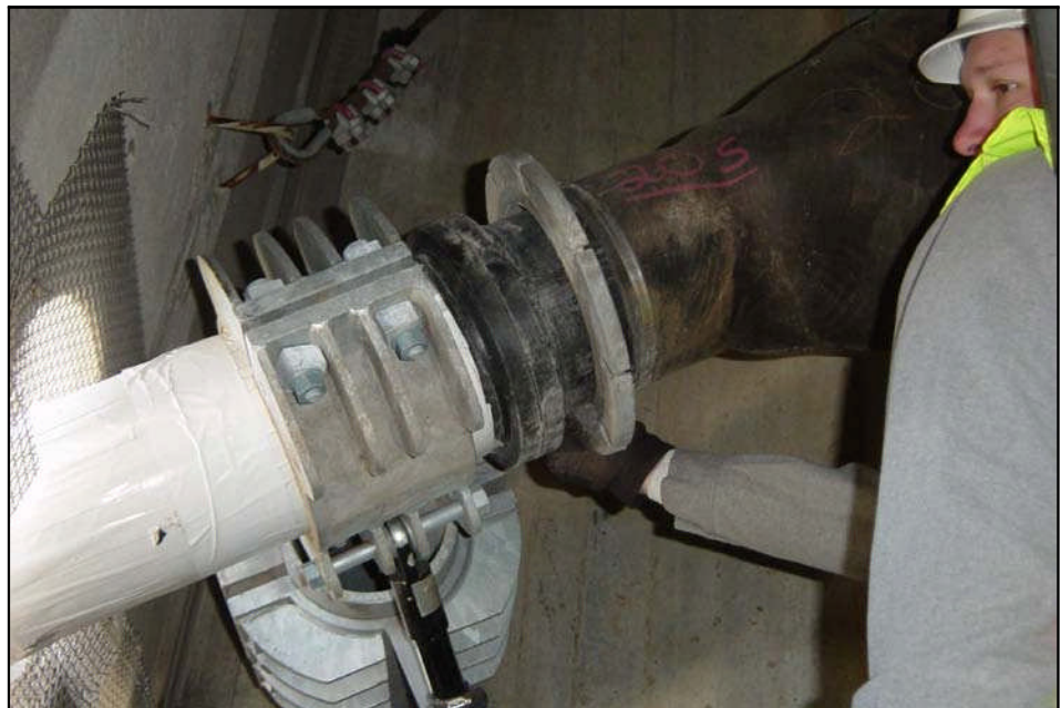
Figure 16.1.35 Damper on Cable-Stayed Bridge
