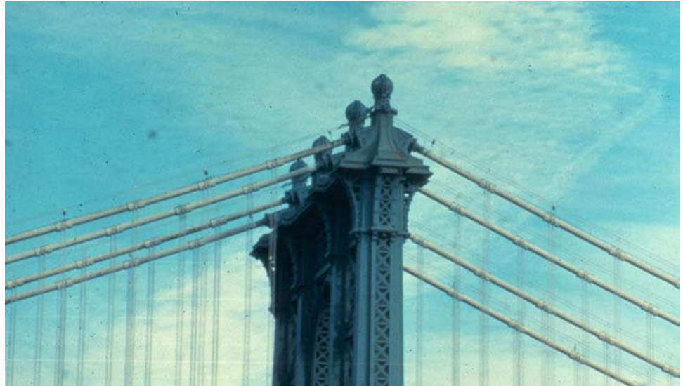
Figure 16.1.18 Cable Saddles for Manhattan Bridge, NYC (Main Span 1,480 ft)
