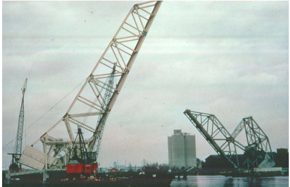
Figure 16.2.32 Concrete Counterweight on a Single-Leaf Bascule Bridge
