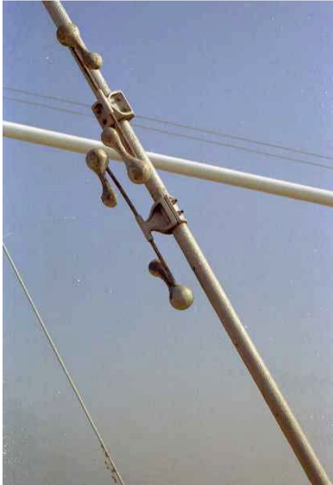
Figure 16.1.51 Tuned Mass Damper System
