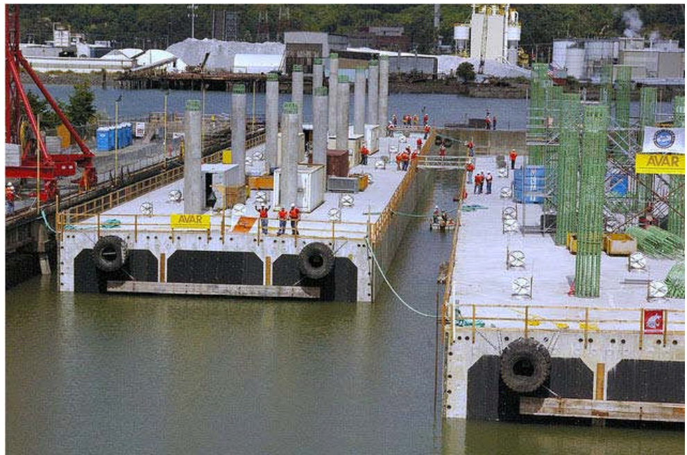
Figure 16.3.6 Concrete Pontoons Transported for Hood Canal Project
