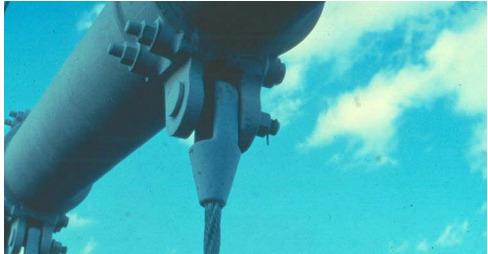
Figure 16.1.20 Open Socket Suspender Cable Connection
