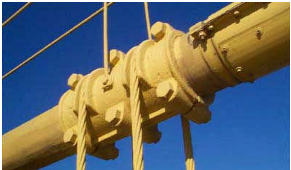
Figure 16.1.19 Grooved Cable Bands
