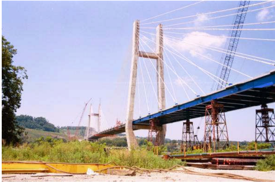
Figure 16.1.2 Maysville Cable-Stay Bridge
