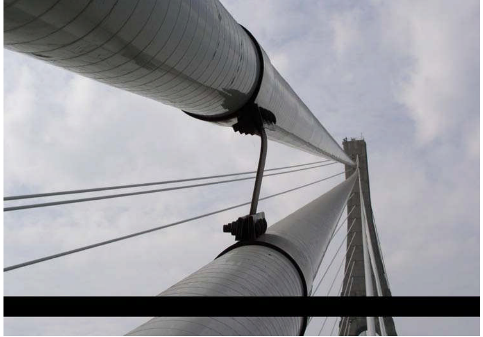
Figure 16.1.50 Cable Tie Type Damper System
