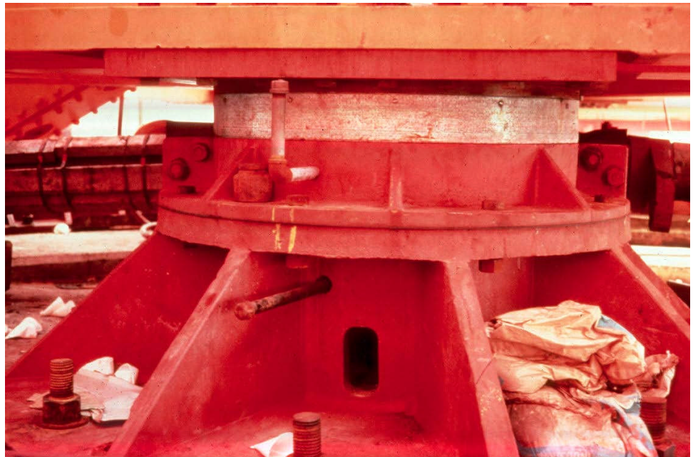
Figure 16.2.36 Center Pivot Bearing
