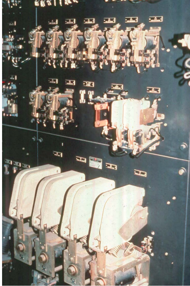
Figure 16.2.65 Open Switchboard
