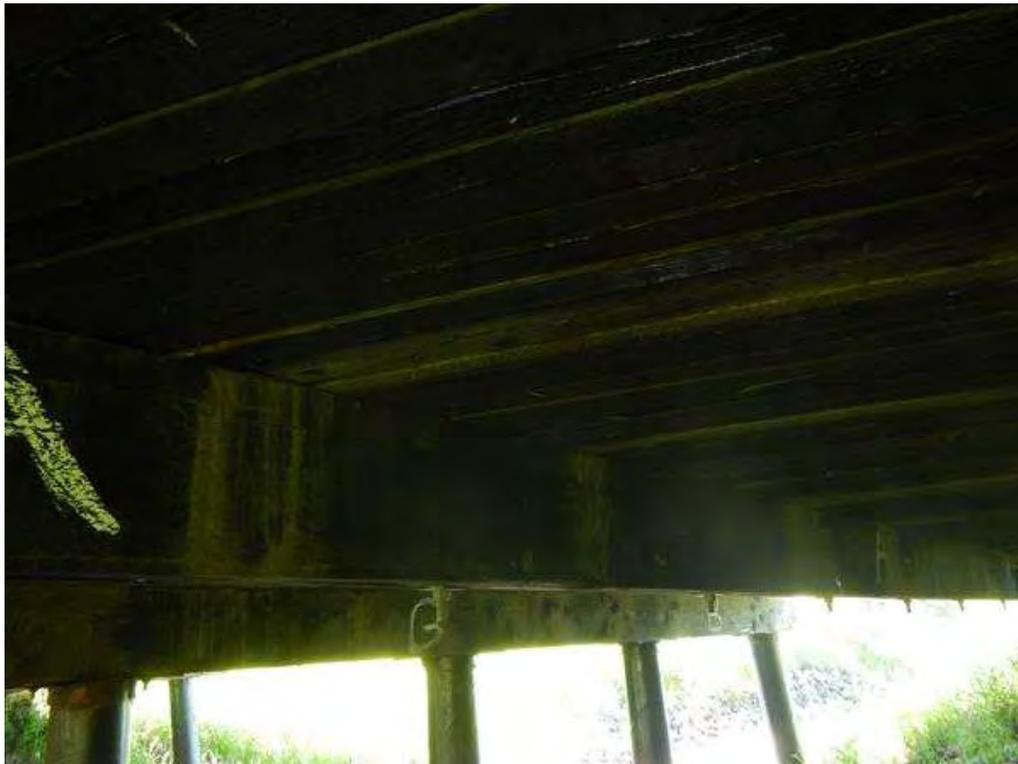
Photo 8 - Span 1 - Moisture pen. through deck.
