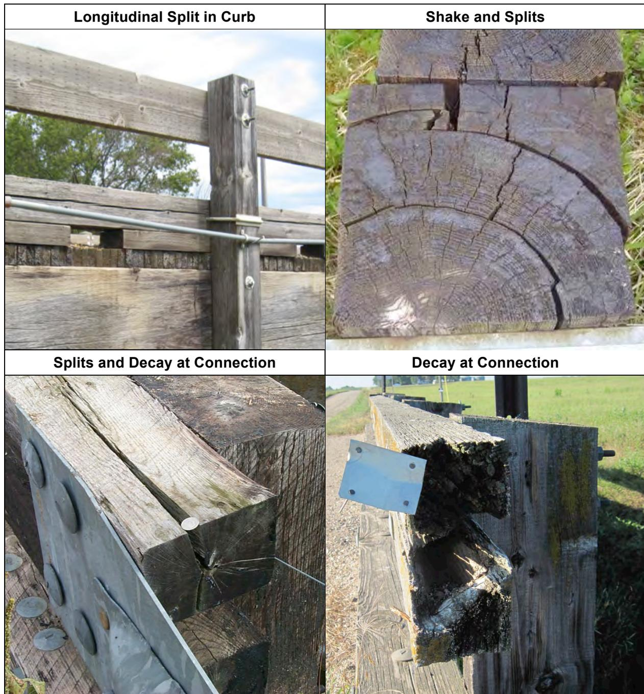
Figure 7.4. Examples of deterioration of timber railing components.
