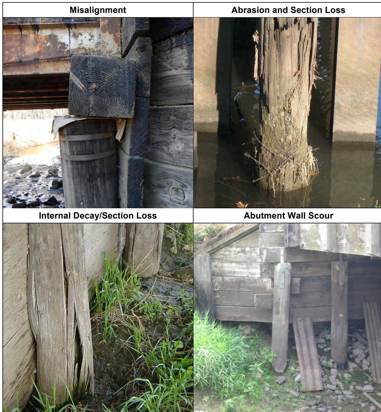
Figure 7.6. Examples of deterioration of timber substructure elements.
