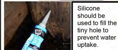
Silicone should be used to fill the tiny hole to prevent water uptake.
