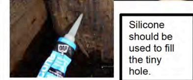
Silicone should be used to fill the tiny hole.
