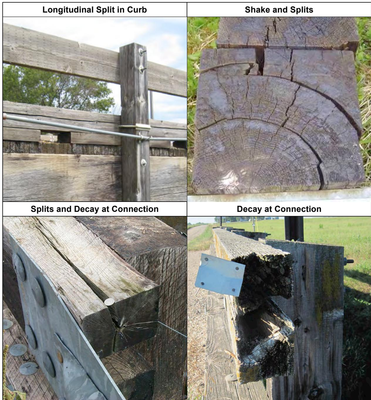
Figure 7.4. Examples of deterioration of timber railing components.
