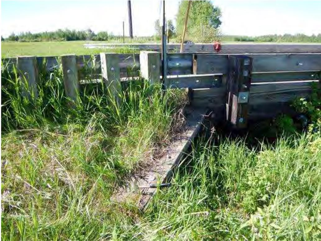
Photo 17 - Wing wall with significant vegetation
