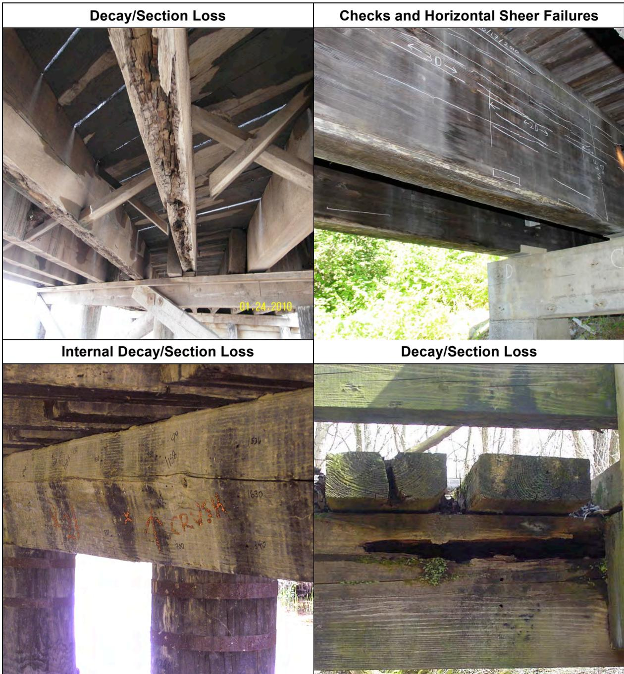
Figure 7.5. Examples of deterioration of timber superstructure elements.
