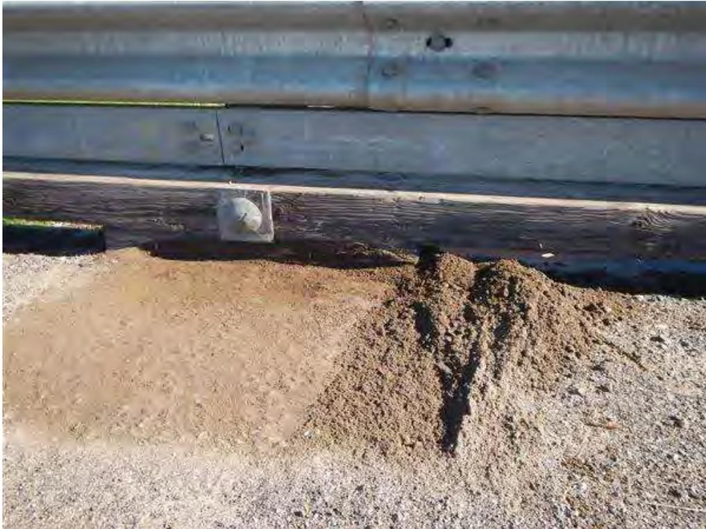
Photo 4 - N. deck-scupper 3" sand on deck
