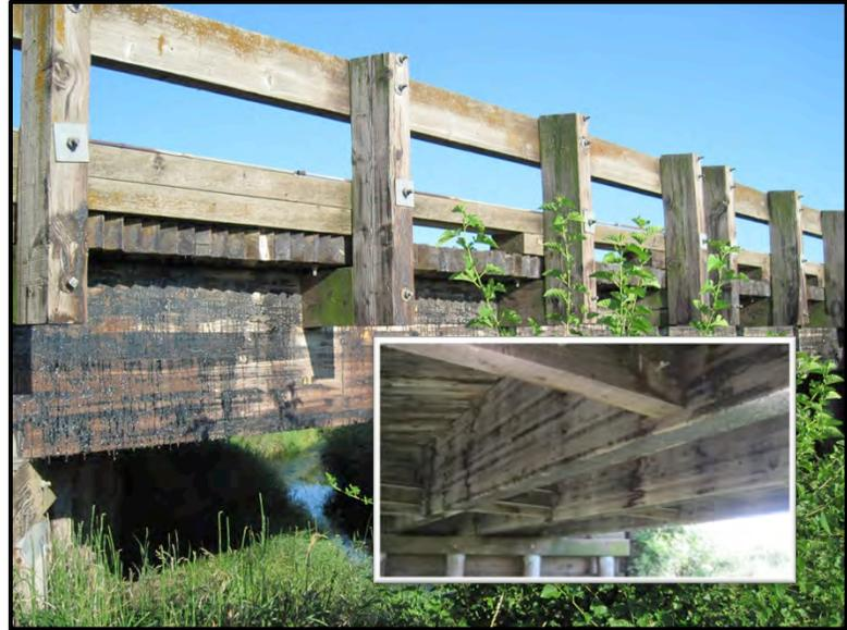
Figure 1.2 Glulam beam timber bridge construction.
