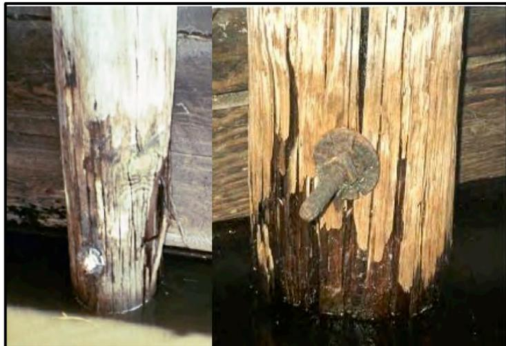
Figure 3.18. Shell damage to timber piling at or near the water line, often caused by freeze thaw cycles, ice damage or flotsam floating down the river.
