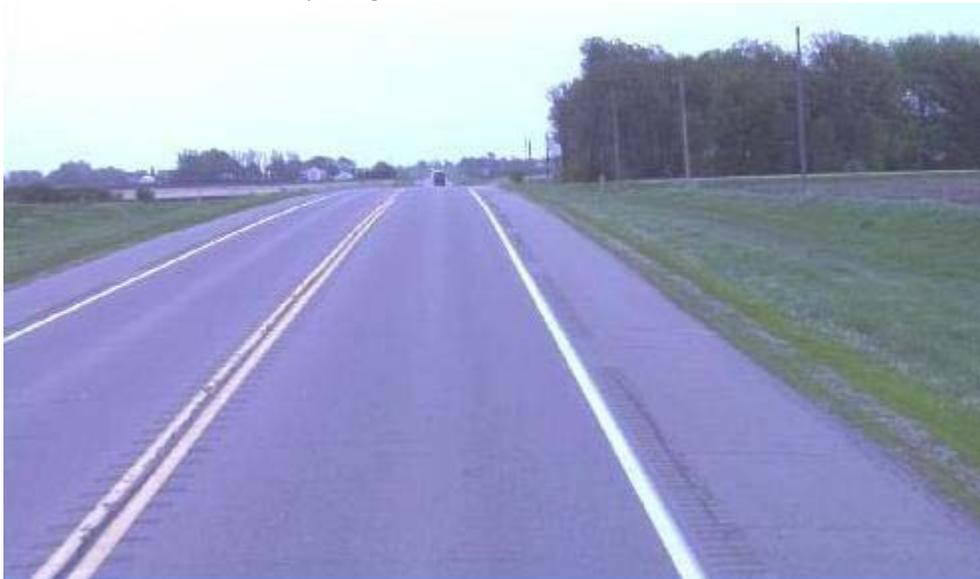
Figure 4 - Shoulder (edgeline) and centerline rumble strips
