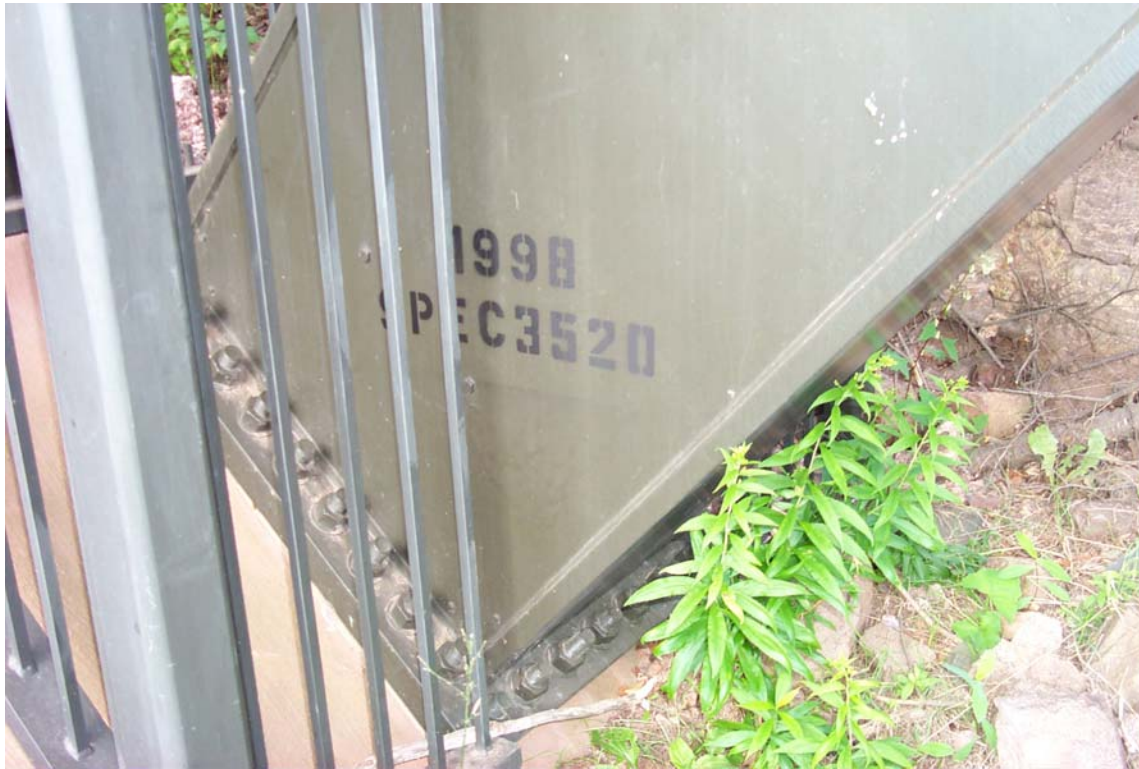
Photo #1: Typical arch footing
