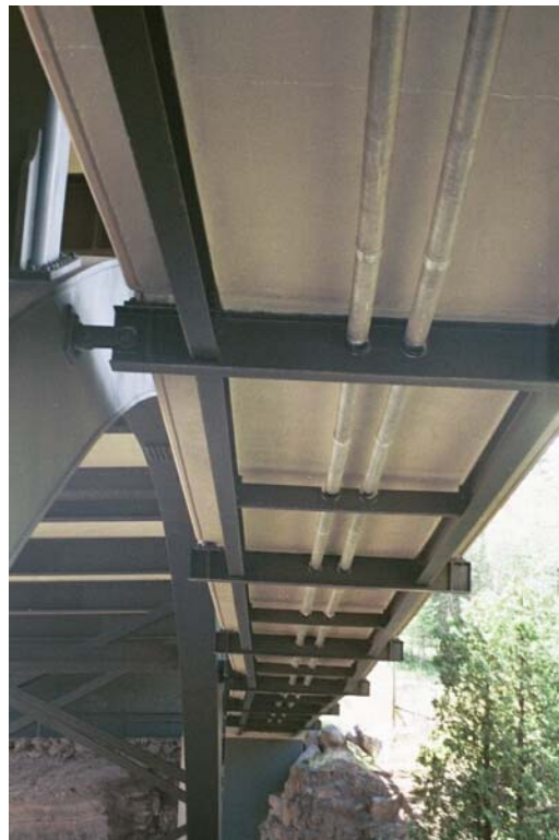
Underside view of sidewalk
