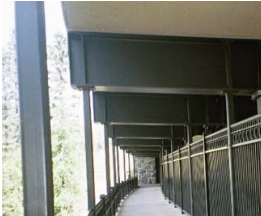
Suspended sidewalk (looking north)
