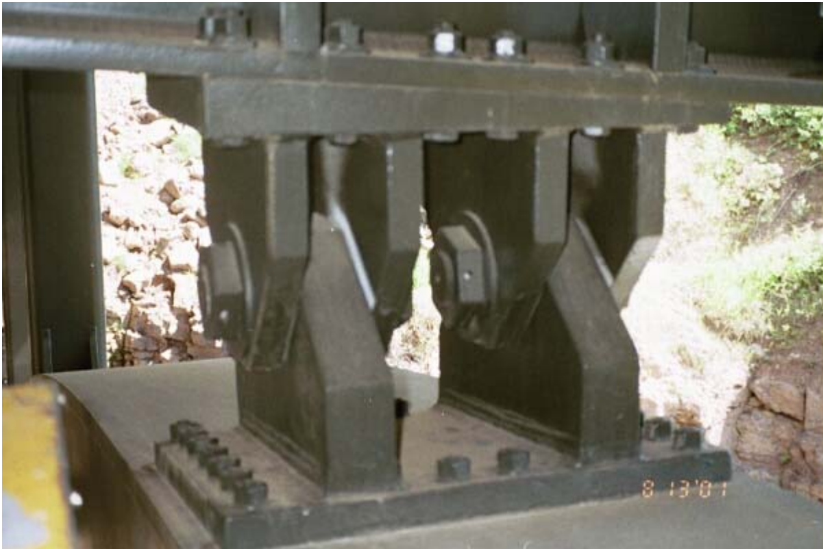
Pinned connection between arch rib & spandrel cap
