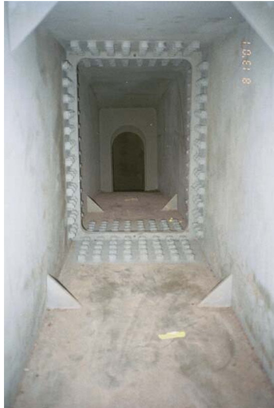
Arch interior - view of splice (top of arch)
