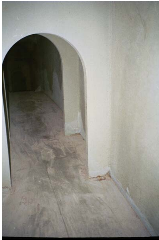
Arch interior - internal stiffeners at spandrel connections
