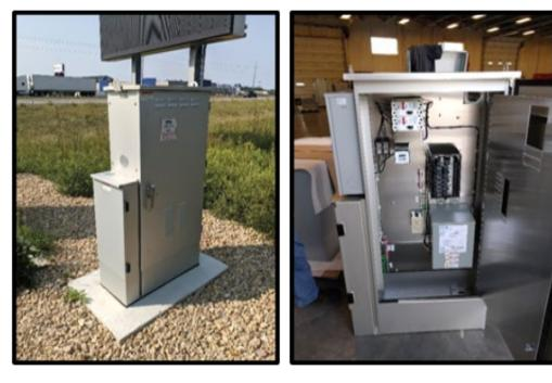
Figure 3-21: Service Cabinet 240/480 with Stepdown Transformer
