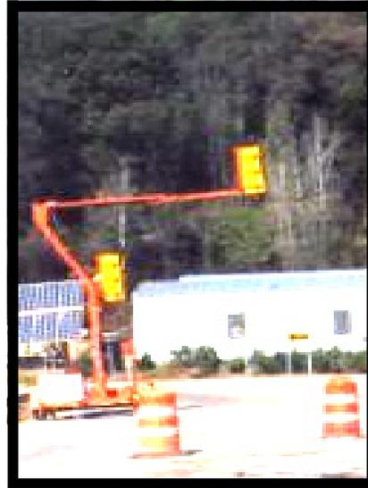
**Purpose:** This project will evaluate the latest solar/battery powered portable traffic lighting for bridge work and maintenance. These units are wireless and improvements in radio communications should make them more reliable. They are able to be set up as far away as one mile from each other and also have the ability to expand to four units.
