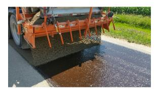
**Project Description:** Chip seals require crews to apply a layer of asphaltic coating on a prepared pavement, followed by spreading small, high-friction aggregate to cover the new pavement surface. Chip spreading machines sometimes fail to evenly spread the high-friction surface rock.
