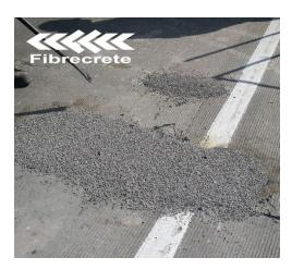
**Project Description:** Crack sealing of concrete pavement can be time consuming and costly. Traditional repairs are prone to failure due to the stiffness of the cement-based sealant. The district is seeking an alternative material that seals cracks as well as cement but which is more durable and lasts longer.
