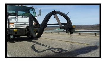
**Project Description:** Heated emulsions used in asphalt pavement repair can easily clog up spray distributors. This results in costly delays and labor to repair and reset equipment. Heated sprayer distributors prevent clogging and provide continuous operation, saving time and money.
