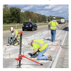
**Project Description:** As part of the 2017 MnROAD construction program under the National Road Research Alliance, researchers identified a section of Interstate 94 in Minnesota that showed damage at concrete pavement joints where loads transfer poorly across 24 slabs in a 600-foot stretch. Joints and the subsurface area require repair before asphalt overlay.
