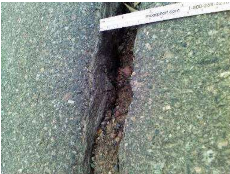
Figure 6 Cell 8011. Crack seal adhesion failure and loss closeup 3/27/20.
