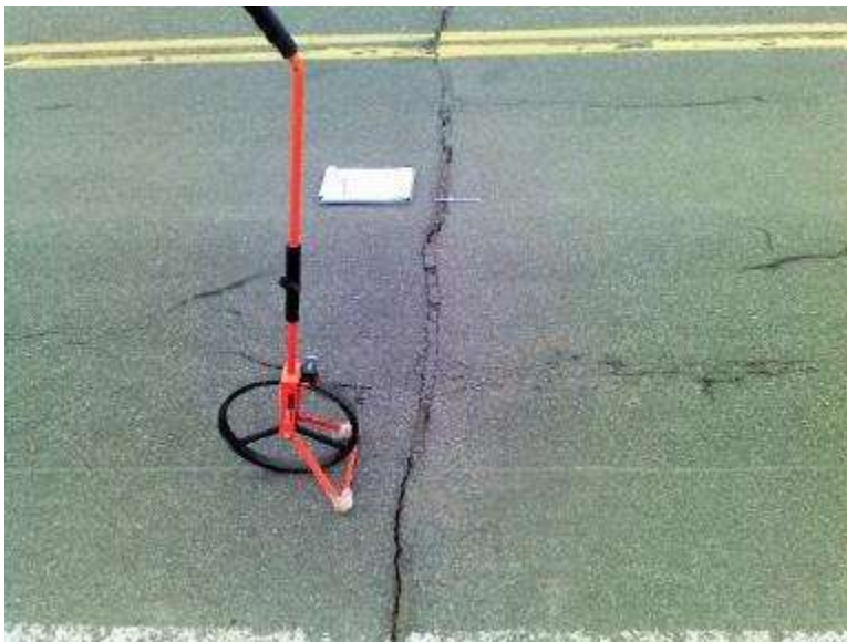
Figure 2 Cell 8011. Crack seal adhesion failure 3/27/20.
