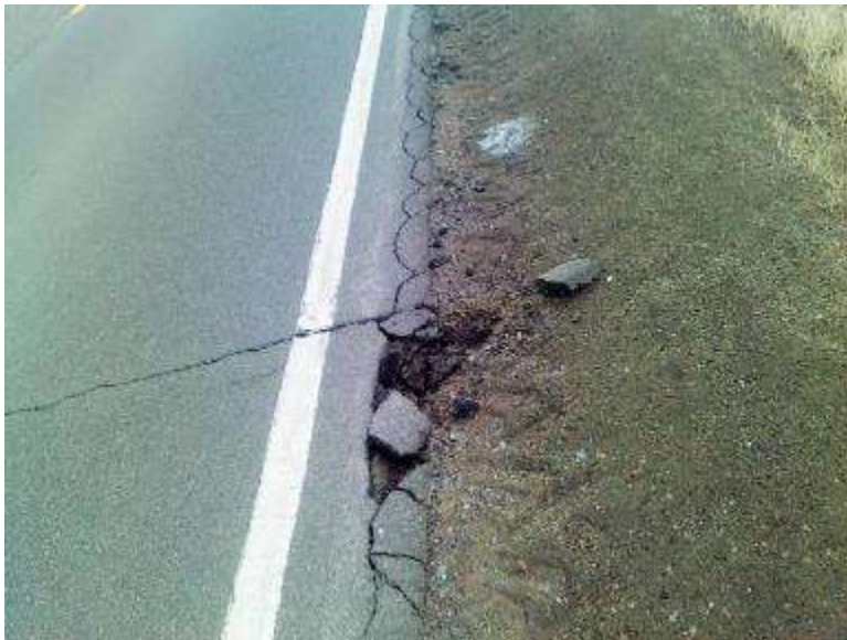
Figure 8 CSAH 8 Thinlay EB. Edge cracking and breakup 3/27/20.
