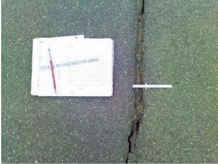
Figure 3 Cell 8011. Crack seal adhesion failure closeup 3/27/20.
