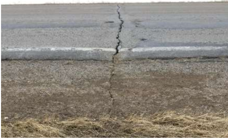
Figure 1 CSAH 8 chip seal section with transverse crack through embankment 2/28/20.
