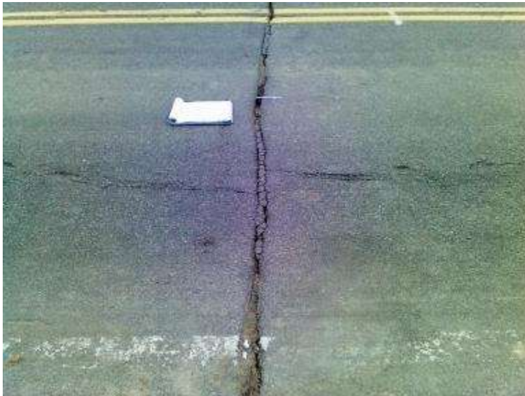
Figure 4 Cell 8011. Crack seal adhesion failure and loss 3/27/20.
