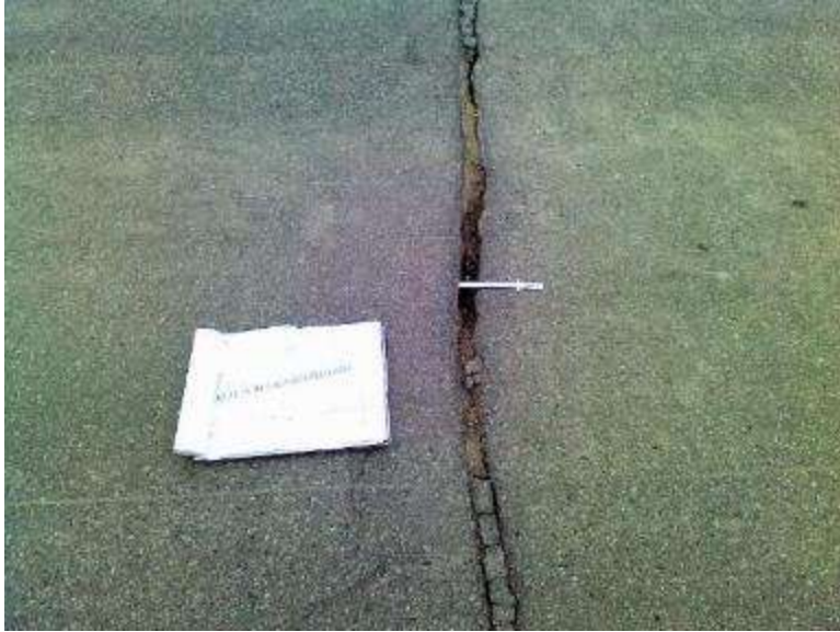
Figure 5 Cell 8011. Crack seal adhesion failure and loss 3/27/20.
