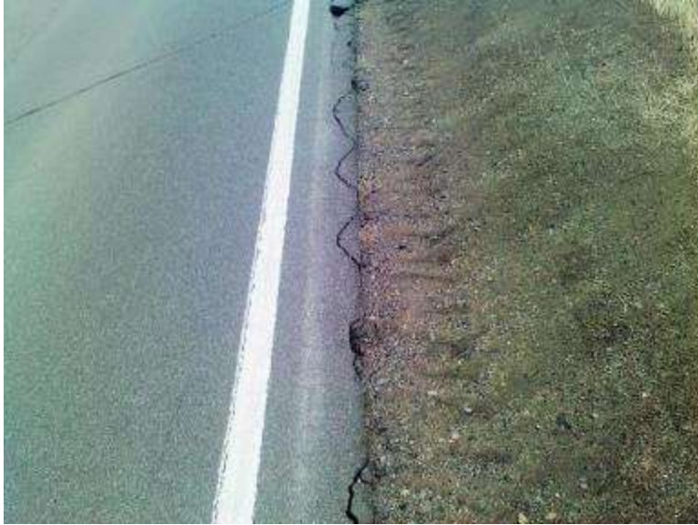
Figure 7 CSAH 8 Thinlay EB. Edge cracking 3/27/20.
