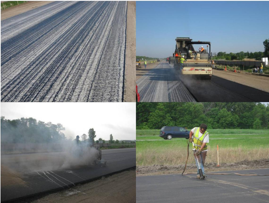
**Figure 6. Tack coat applied to PCC surface (top left) prior to HMA paving (top right). Sawing (bottom left) and sealing (bottom right) HMA layer – saw cuts in the HMA were matched to the saw cuts in the PCC below to within 12.5 mm (0.5 in)**
