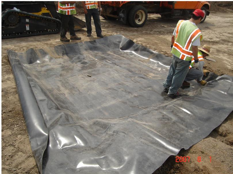
**Installation of Lysimeter to Collect Leachates from Base Materials**
