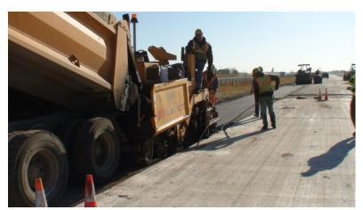
Figure 5.6. MnROAD MWSS Shoulder Construction
