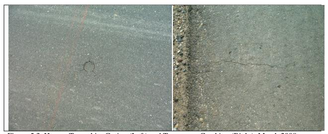
Figure 5.3. Hassan Township: Coring (Left) and Transverse Cracking (Right), March 2008
