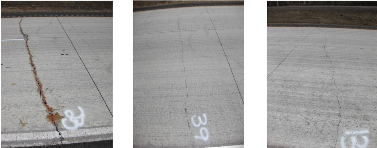
Figure 5.2. From Left to Right: High (3), Medium (2) and Low (1) Severity Cracking
