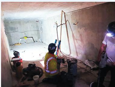
Following bridge inspections, about one-third of discovered grout voids were filled using vacuum-assisted or pressure grouting repair techniques.
