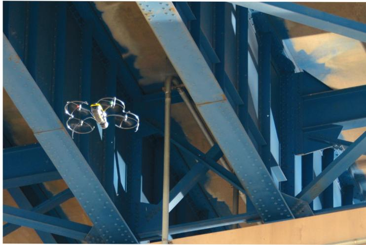
This senseFly drone accesses under-deck locations that are difficult or impossible to reach with ropes or snoopers.
