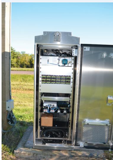
Roadside WIM cabinets contain equipment that captures information on vehicle counts, speed, and axle weights and distribution.
