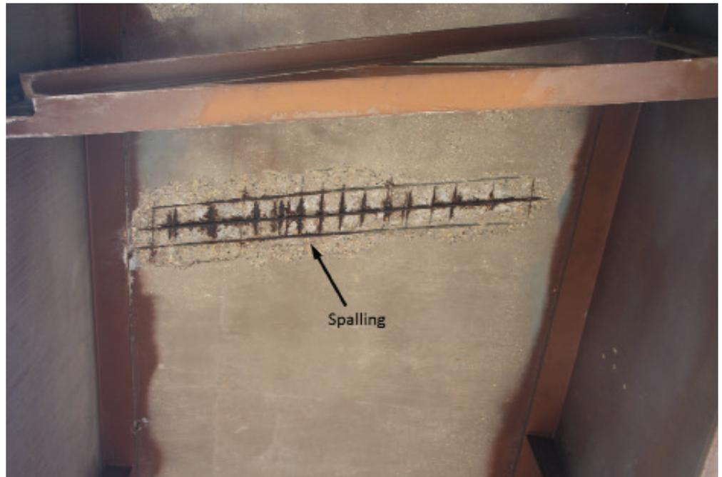
Spalling has occurred because deicing chemicals and water have seeped into the concrete deck through cracks in the deck surface, causing uncoated steel reinforcement to corrode and concrete to spall.
