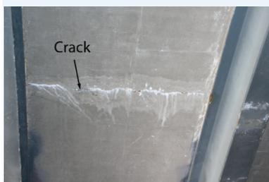
Cracks on the undersides of a bridge deck can leak as chlorides corrode steel and seep through the crack.
