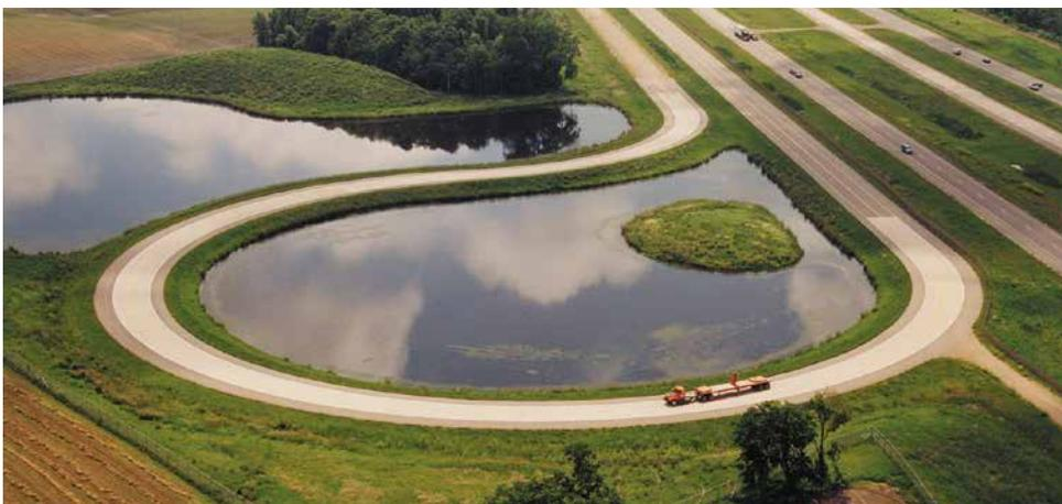
MnROAD's facility includes a test section of I-94 carrying live traffic, a low-volume roadway that simulates rural road conditions, and thousands of sensors that record load response and environmental data.
