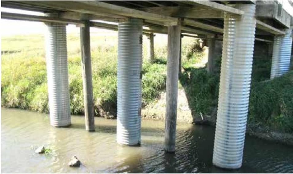
One of the timber bridge rehabilitation procedures detailed in the manual involves concrete pile jackets, which are concrete-filled steel shells installed to strengthen timber piles.
