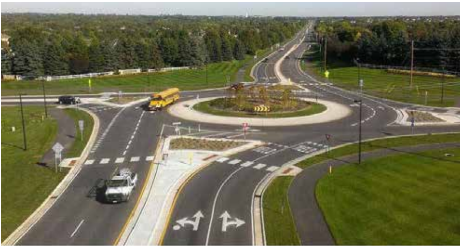
Reductions in speed associated with speed control treatments will decrease the likelihood of crashes as drivers approach and enter roundabouts.
