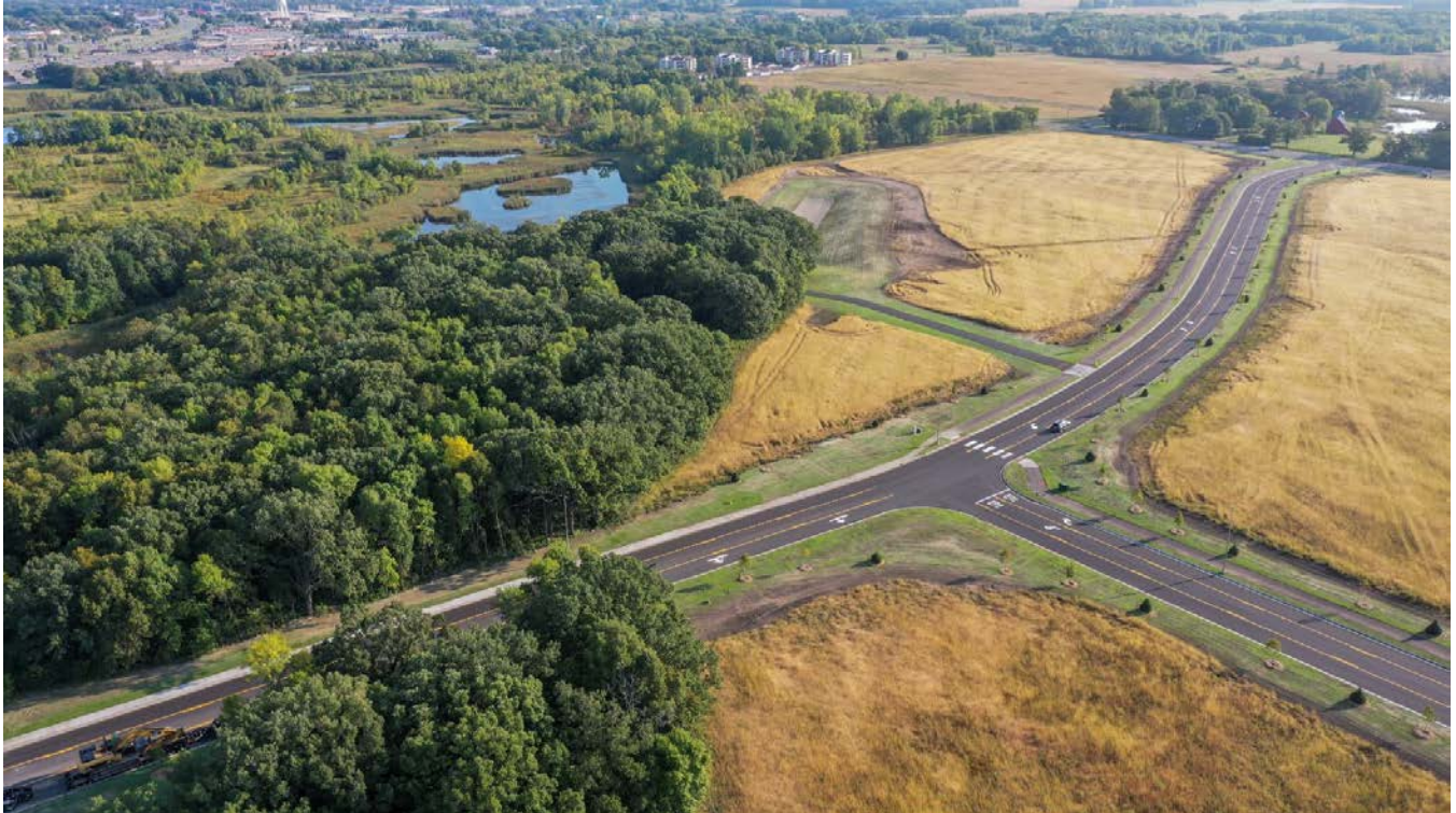
Alexandria 44th Avenue project
