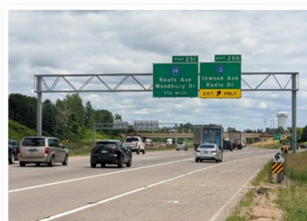
Sign Bridge (Design D) (current design)
