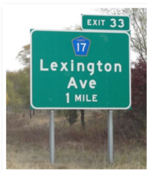
I-beam Sign (with exit number panel)
