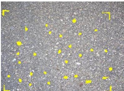
Weathering – At low severity, the coarse aggregate is slightly exposed due to the wearing away of the fine aggregate. At medium severity, the coarse aggregate is exposed up to ¼ the width of the longest side. At high severity, the coarse is exposed greater than ¼ the width of the longest side.
