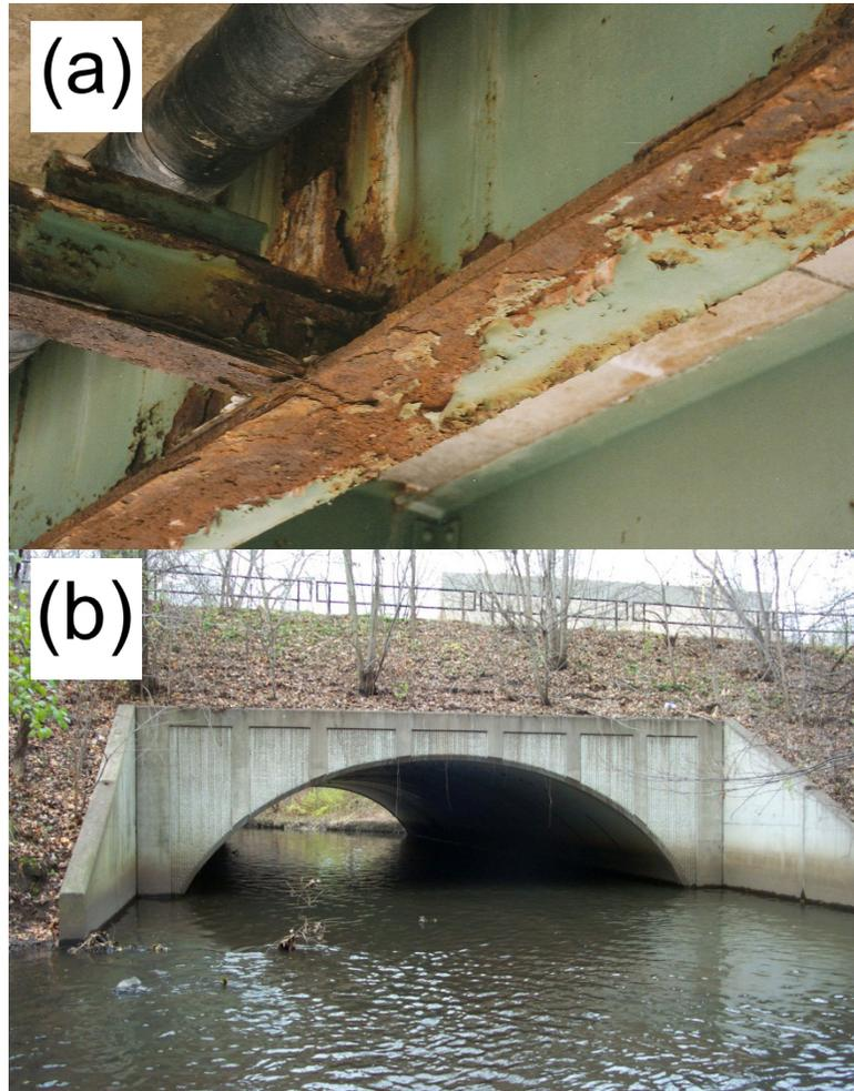
Culverts [see [Figure 6-6 \(b\)](#)] tend to be more durable due to the fact that they are generally protected underground and are manufactured under more controlled conditions. They also deteriorate, but at a slower rate than bridges.
