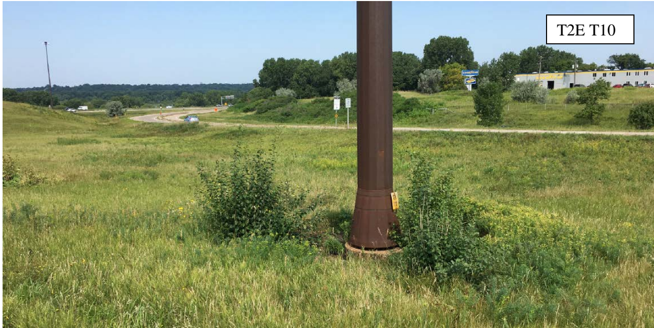
Figure 3: T2E T10 is the most preferred location, from an access and safety perspective; it is along MN 13, where traffic is lighter and the location is well off both the mainline and the ramp. The ground is relatively flat for good CPT truck access.
