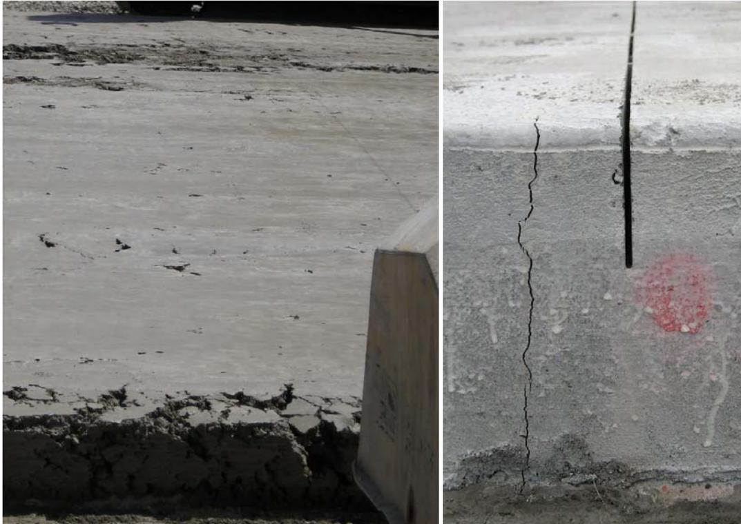
11 **Figure 3. At left, “torn” edges and surface due to concrete setting on profile pan; at right,**
