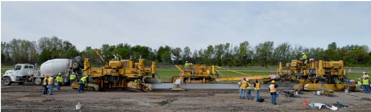
**Figure 2. Paving train constructing R21 research sections along I-94 at MnROAD (from left to right, the mixer truck, first paver, material transfer device, and second paver)**
