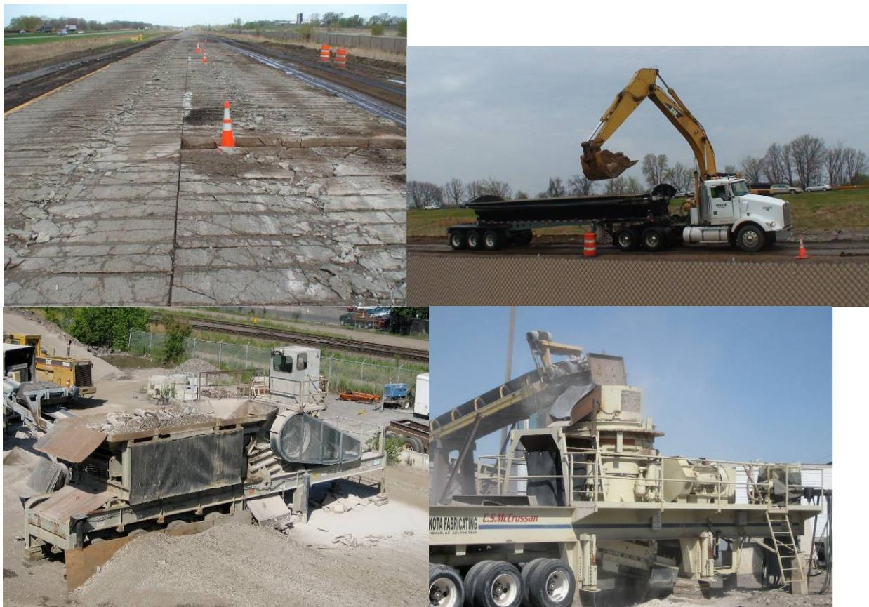
**Figure 1. Salvage operations showing broken PCC pavement (top left) and removal (top right). Jaw crusher (bottom left) and cone crusher (bottom right) used in the production of RCA at MnROAD**
