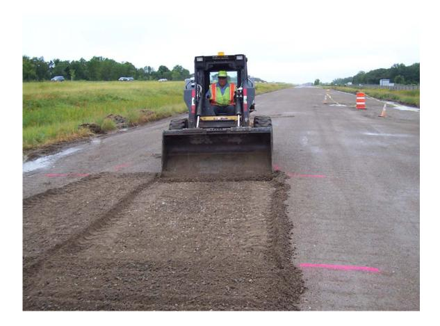
Fig. A-1. Preparing indentation in sub-base for lysimeter geomembrane.
