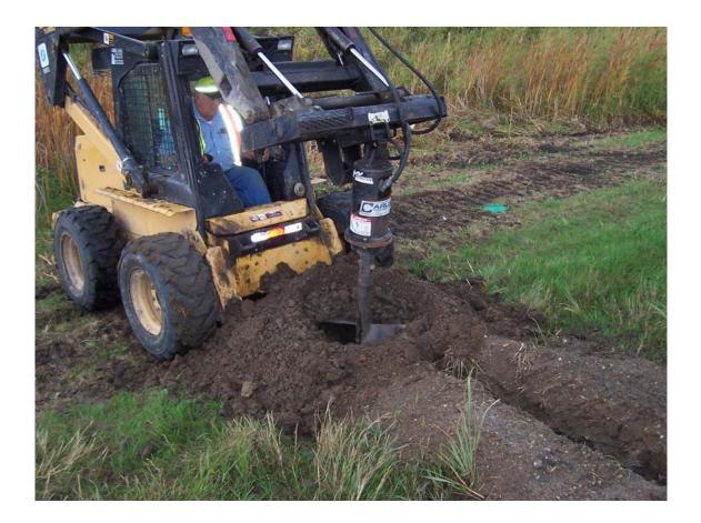
Fig. A-5. Preparing hole for leachate collection tank and trench for drainage pipe.
