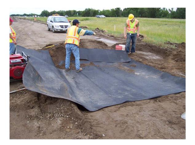
Fig. A-3. Installing geomembrane for lysimeter.
