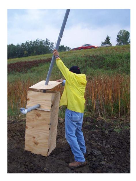
Fig. A-6. Assembling leachate collection tank.
