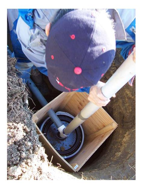
Fig. A-7. Installing leachate collection tank.
