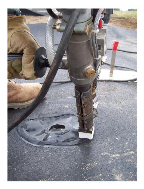
Fig. A-4. Welding geomembrane to lysimeter drainage pipe assembly.
