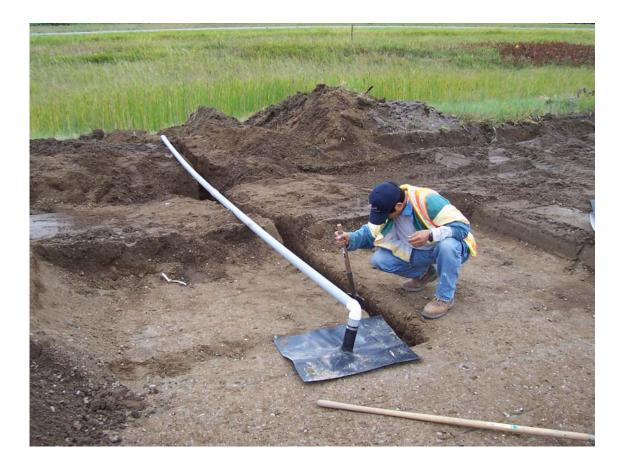
Fig. A-2. Preparing drainage pipe from lysimeter to collection tank.
