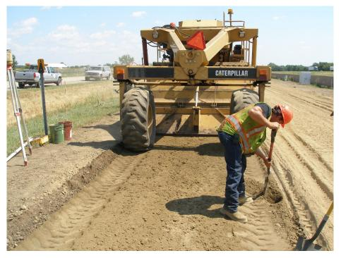
Figure 3. Placement and Mixing of Fly Ash
