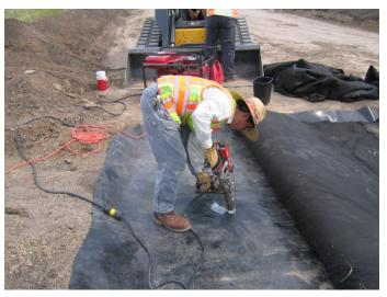
Figure 2. Installation of Lysimeter
