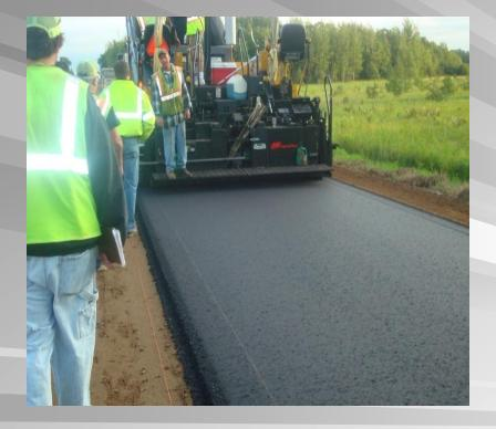
Crow-Wing Co. has used PG58-28 WMA as an Alternate to PG58-34 HMA
