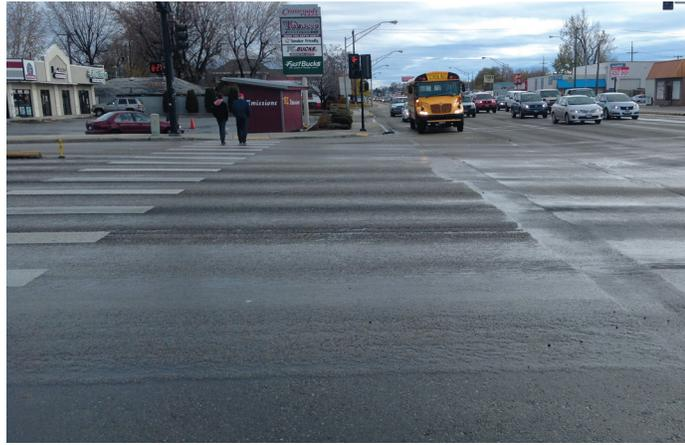
Rutted and otherwise damaged asphalt pavement is a candidate for a bonded concrete overlay that can mitigate damage under the right site conditions.
