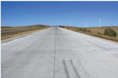
Done well, whitetopping of asphalt pavement extends pavement life for decades.
