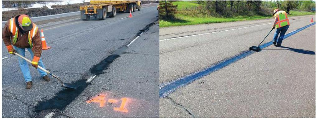
(Left) A road worker tamps cold-mix asphalt into a pothole along a shoulder joint on Highway 61 north of Duluth. (Right) Another worker levels off mastic material filling a longitudinal crack on Interstate 35.
