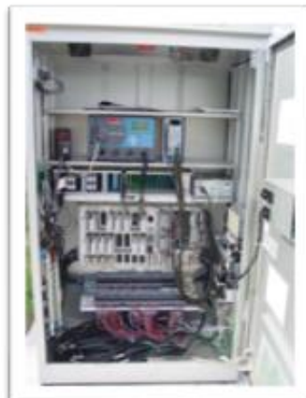
Right: Interior of signal service cabinet
